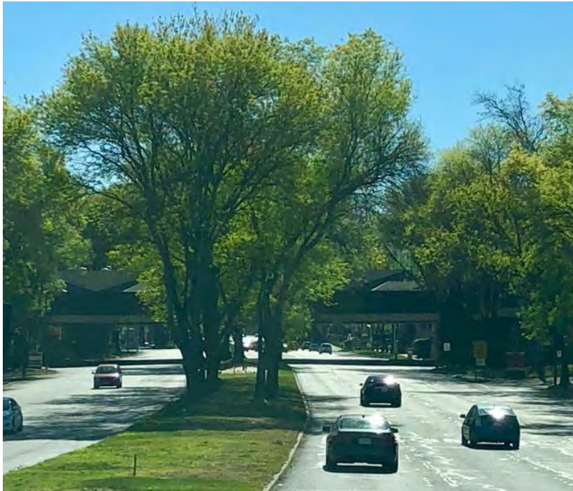
Figure 12: SB Wolfe Rd.
