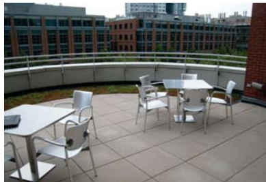
Concrete roof paver system
