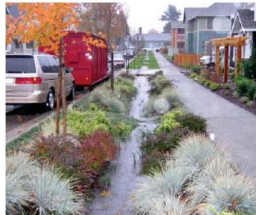
Flow-through curbside rain gardens
