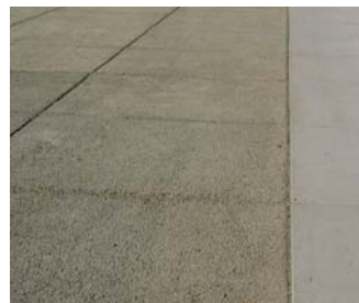
Porous Concrete at parking stalls, where feasible
