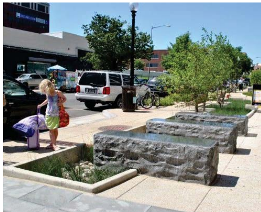
Rain gardens and flow through planters integrated with Pedestrian environment
