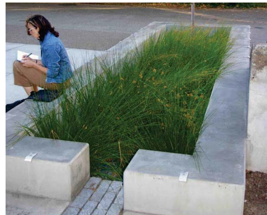
Seat walls at curbside rain gardens
