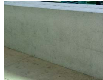
Cast-in-place concrete walls
