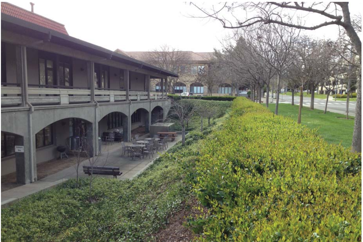
PHOTO 2: View of the existing City Hall building and landscaping on-site from the parking lot looking west.
