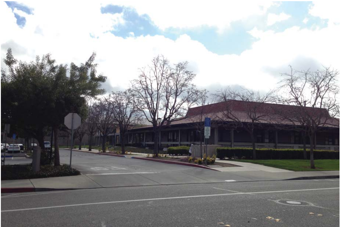
PHOTO 1: View of the existing City Hall building, Rodrigues Avenue, and the Rodrigues Avenue driveway from Rodrigues Avenue looking south.
