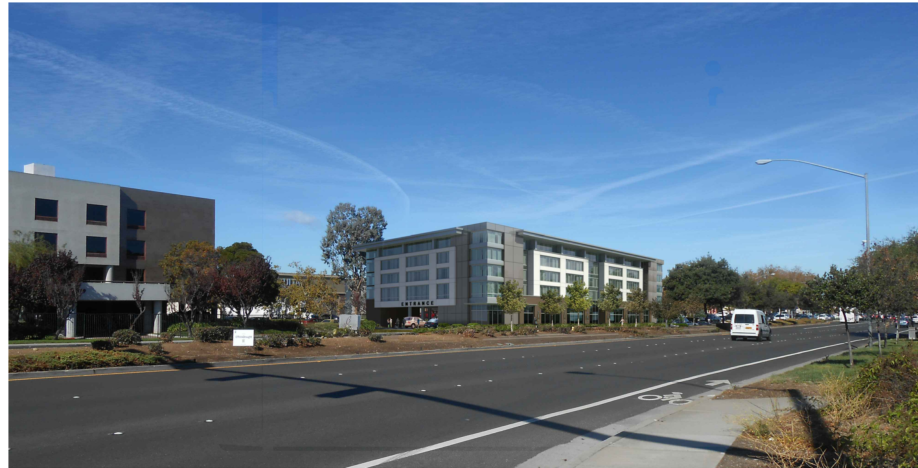
VIEW FROM SOUTH EAST CORNER
