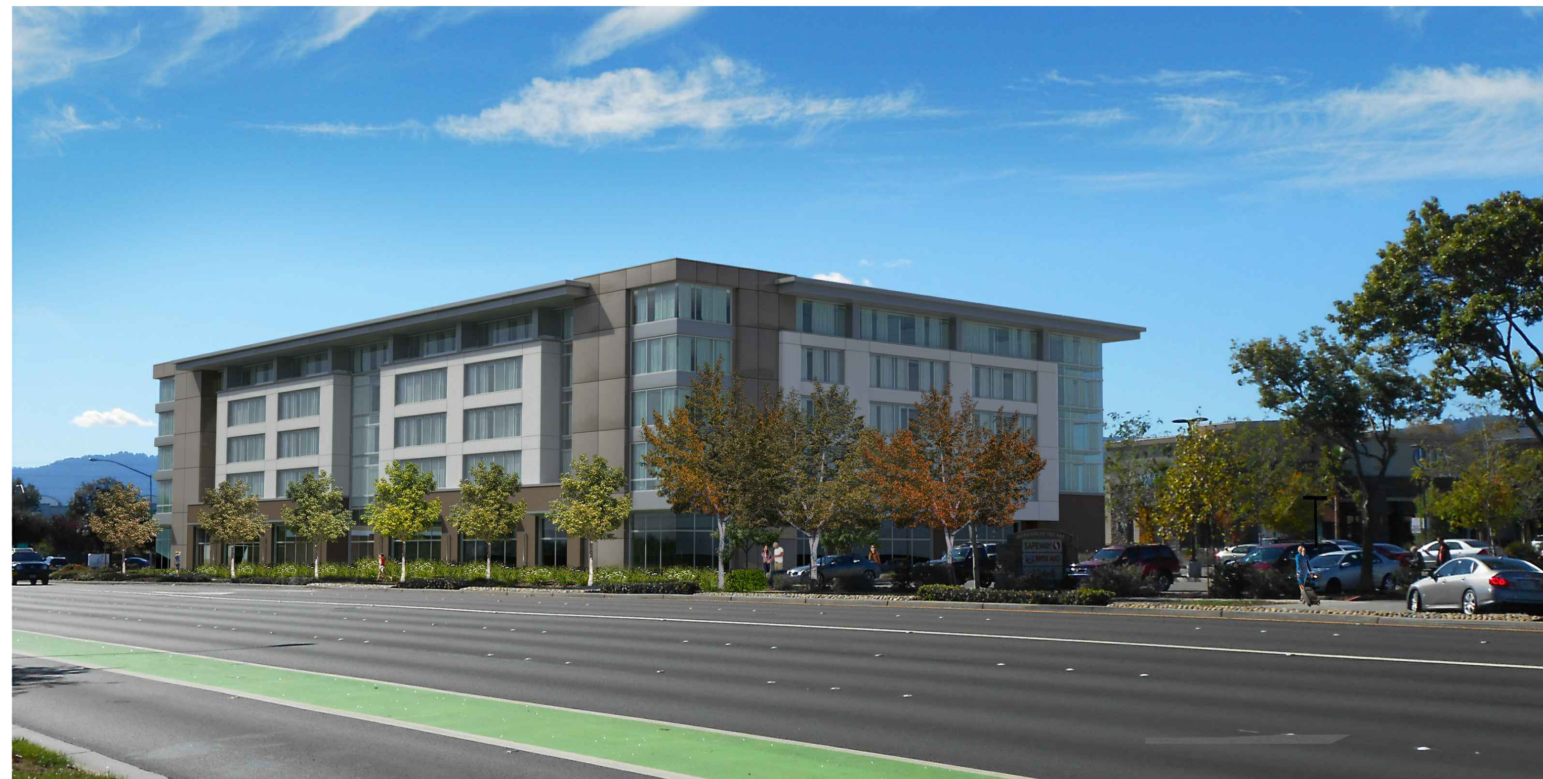
VIEW FROM NORTH EAST CORNER
