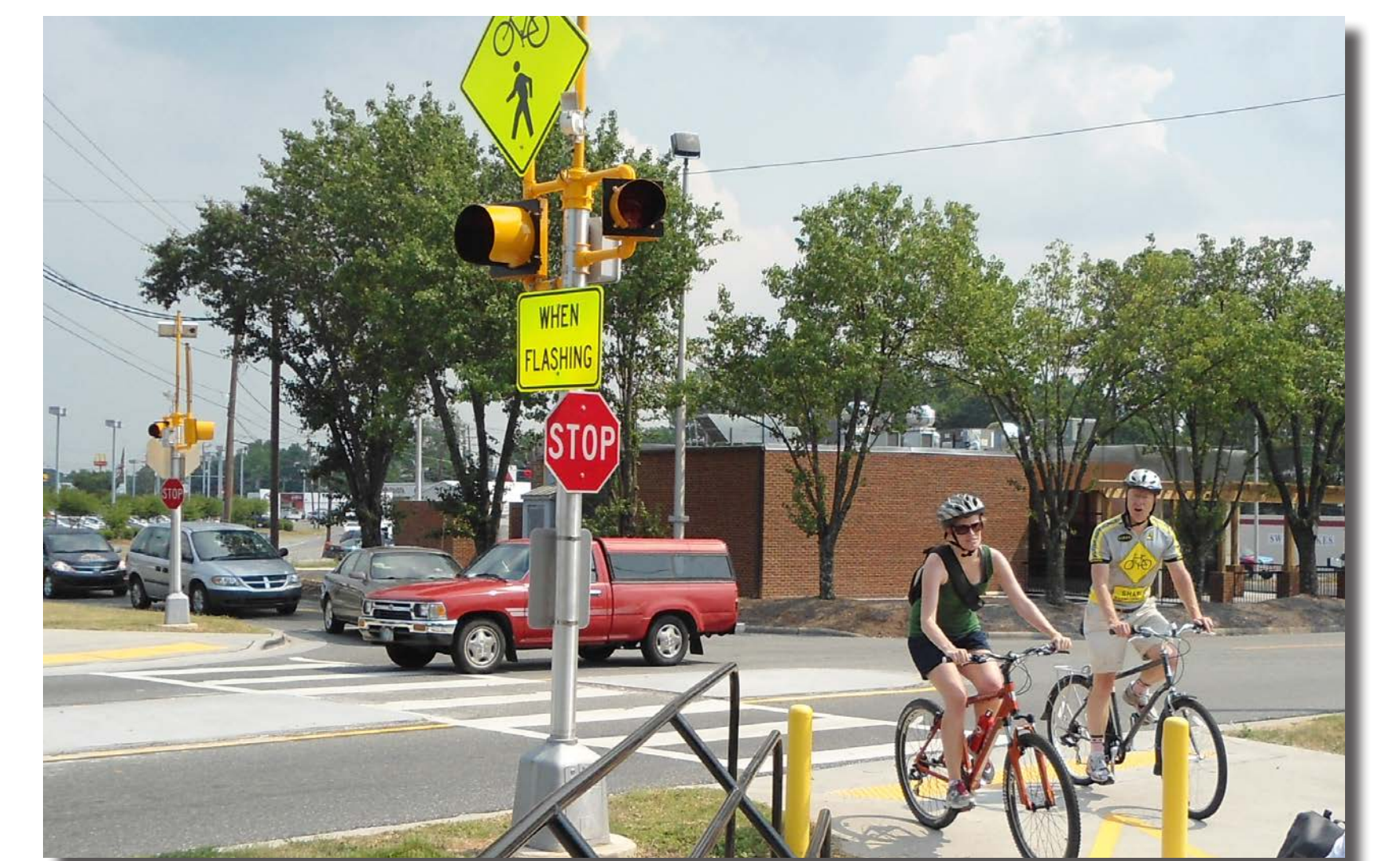
Enhanced crosswalk with beacon
