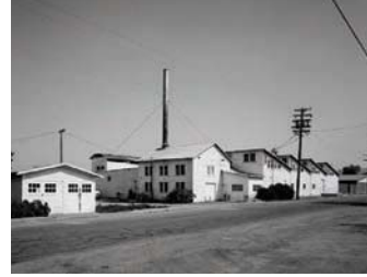
Woelffel Cannery 10120 Imperial Avenue Demolished
