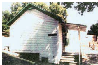
Montebello School 15101 Montebello Road
