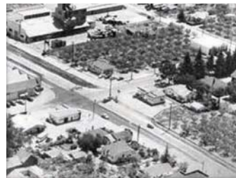
The Crossroads Intersection at Stevens Creek Boulevard and De Anza Boulevard
