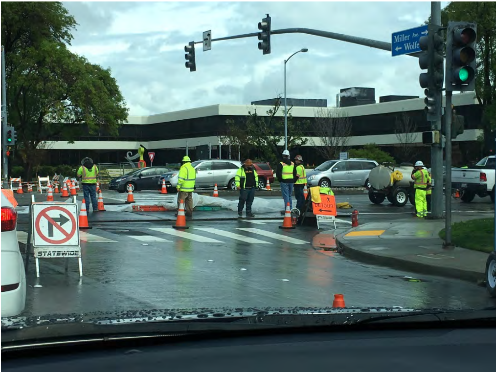
Months of disruptive trenching on Wolfe Road for Apple Park:
