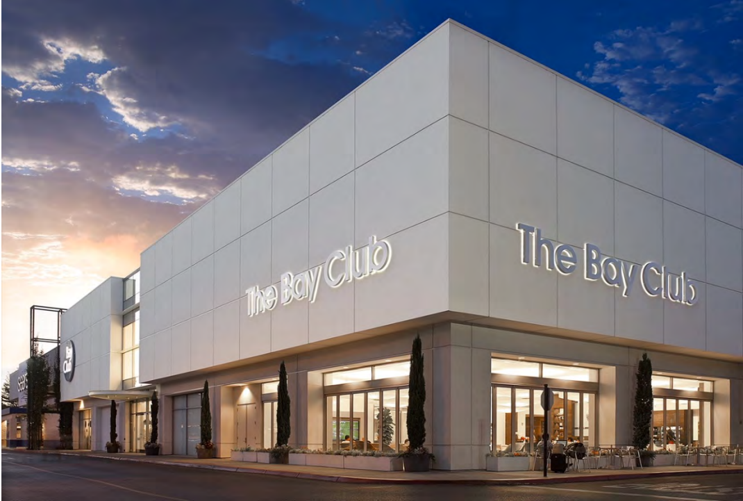
Remodeled three level Bay Club and Starbucks with large gathering room in Sears' building
