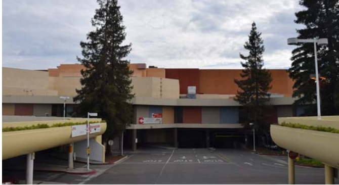
Figure 1.3. Vallco Mall, view from an interior parking court.
