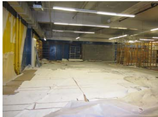
Photograph 26. Former auto service area at JC Penney.
