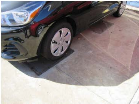
Photograph 25. Steel covers to oil/water separator at SAC.
