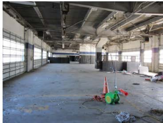
Photograph 16. Interior of SAC building.
