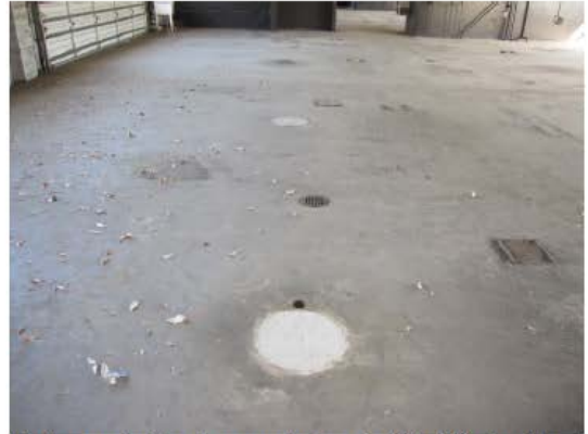
Photograph 18. Former hydraulic lifts (filled with concrete) at SAC.
