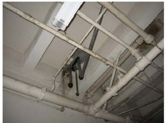
Photograph 22. Remnant hydraulic lift piping (unpainted) in basement at SAC.
