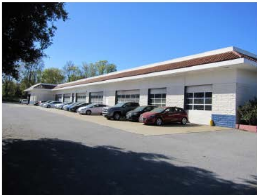
Photograph 15. Sears Automotive Center (SAC) building.
