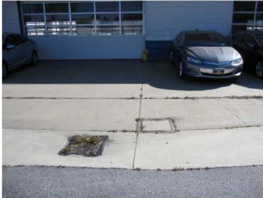
Photograph 23. Concrete access cover (near storm drain) at the suspected waste oil UST location at SAC.
