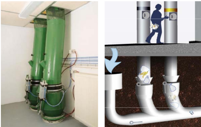
Diagram 1.4.2.2 – Example of Pneumatic Waste System Valve Room
