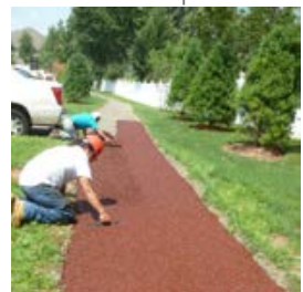
Porous pavement path
