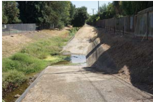
Photo 3.15: Maintenance access ramp
