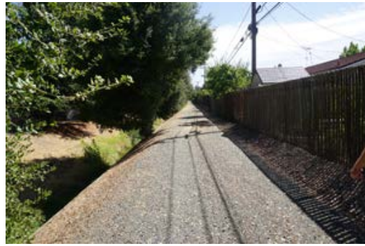
Photo 3.13: Regnart Creek maintenance access road
