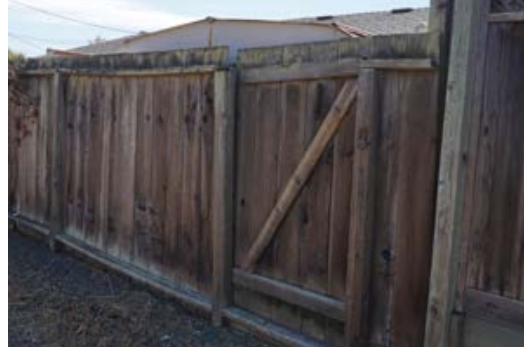
Photo 3.14: Residential fencing along creek maintenance road
