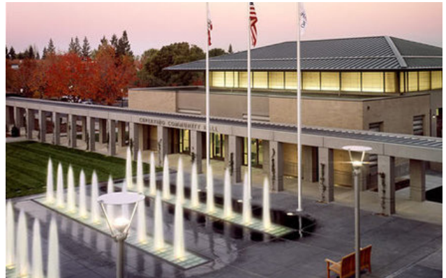
Photo 3.6: Cupertino City Hall
