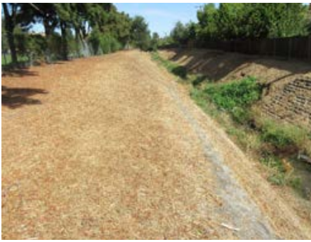
Photo 1: View of the SCVWD maintenance road, on which the trail is proposed to be placed, looking north with residences located on the east side of the creek (to the right). Cupertino City Hall & Library are located to the left (west).
