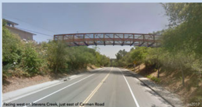
Facing west on Stevens Creek, just east of Carmen Road
