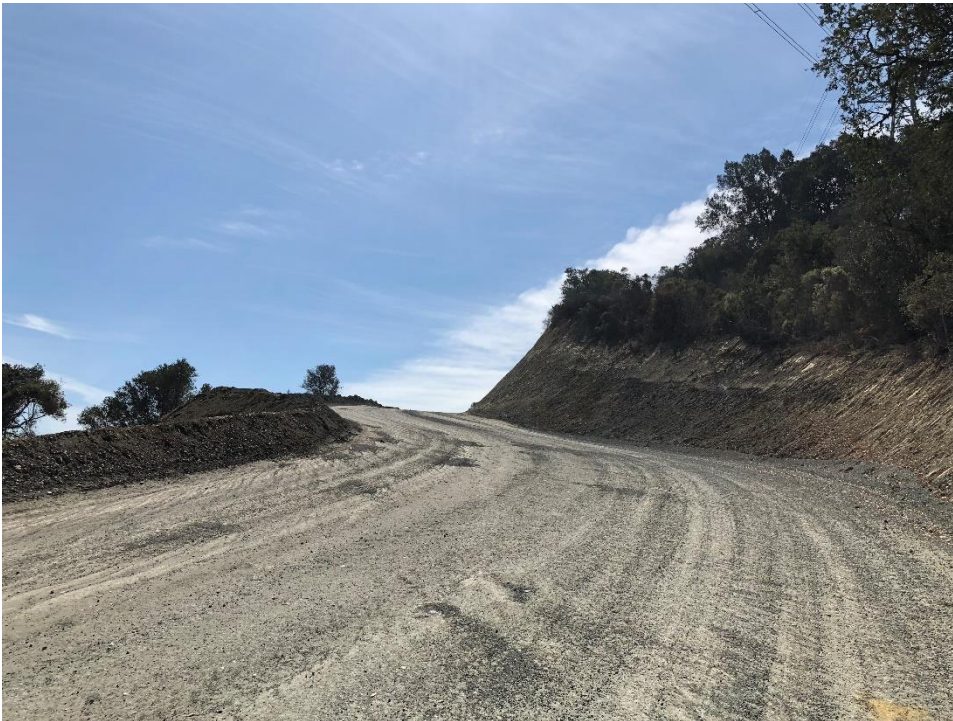
View to the north along the improved existing access road.
