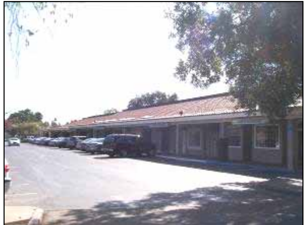
4. North (front) façade of Building F
