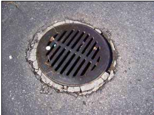
7. Storm drain inlet
