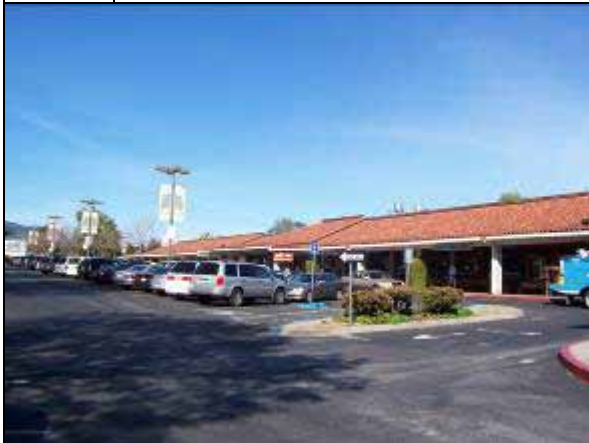
3. South (front) façade of Buildings C and D
