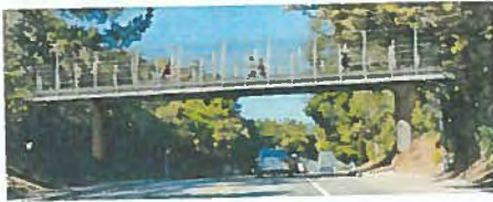
Option 1: Steel Girder Bridge
