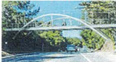
Option 5: Steel Inclined Arch Bridge
