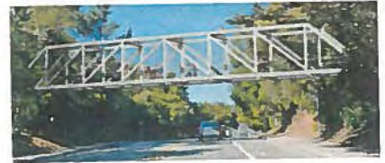
Option 3: Steel Howe Truss Bridge
