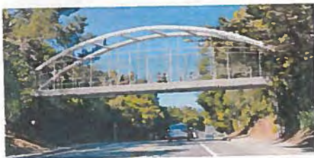
Option 4: Steel Tied Arch Bridge
