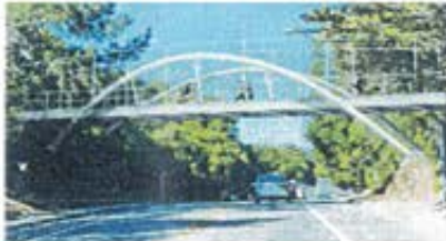
Option 5: Steel Inclined Arch Bridge
