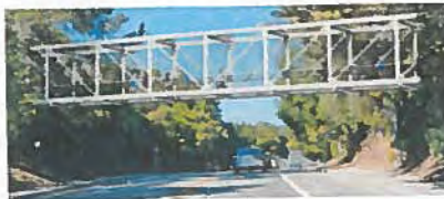
Option 2: Steel Pratt Truss Bridge
