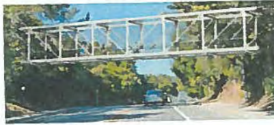
Option 2: Steel Pratt Truss Bridge
