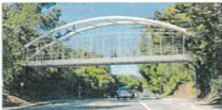
Option 4: Steel Tied Arch Bridge
