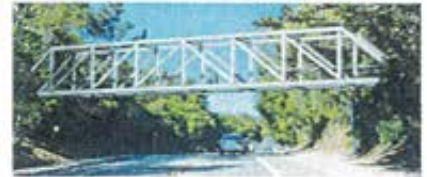
Option 3: Steel Howe Truss Bridge
