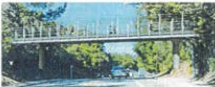
Option 1: Steel Girder Bridge
