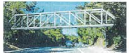
Option 3: Steel Howe Truss Bridge
