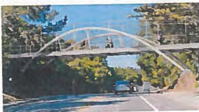
Option 5: Steel Inclined Arch Bridge
