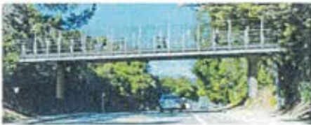
Option 1: Steel Girder Bridge
