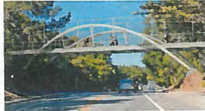
Option 5: Steel Inclined Arch Bridge
