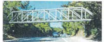
Option 3: Steel Howe Truss Bridge
