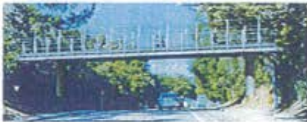
Option 1: Steel Girder Bridge
