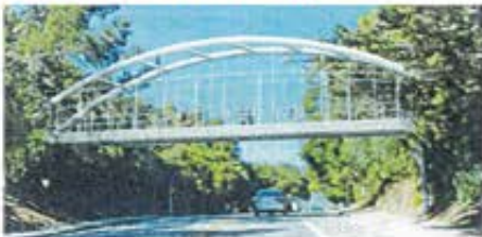
Option 4: Steel Tied Arch Bridge
