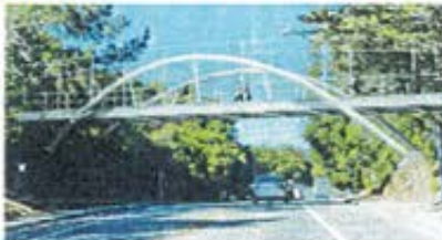
Option 5: Steel Inclined Arch Bridge
