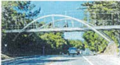
Option 5: Steel Inclined Arch Bridge
