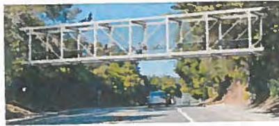
Option 2: Steel Pratt Truss Bridge
