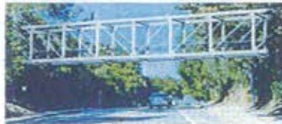
Option 2: Steel Pratt Truss Bridge
