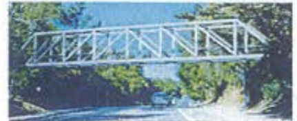
Option 3: Steel Howe Truss Bridge
