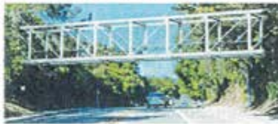
Option 2: Steel Pratt Truss Bridge
