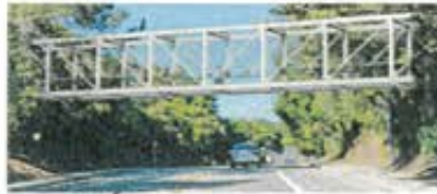
Option 2: Steel Pratt Truss Bridge
