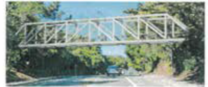
Option 3: Steel Howe Truss Bridge
