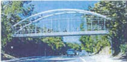
Option 4: Steel Tied Arch Bridge
