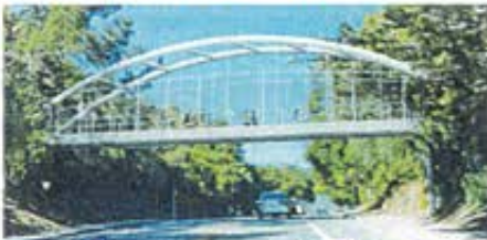
Option 4: Steel Tied Arch Bridge
