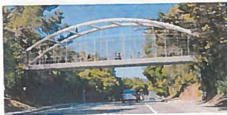
Option 4: Steel Tied Arch Bridge
