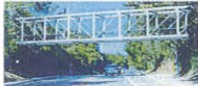
Option 2: Steel Pratt Truss Bridge
