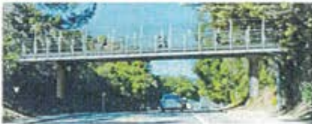
Option 1: Steel Girder Bridge
