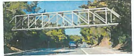
Option 3: Steel Howe Truss Bridge
