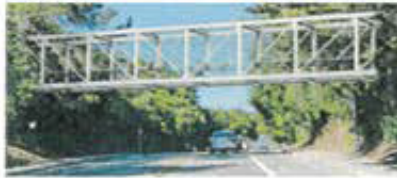
Option 2: Steel Pratt Truss Bridge
