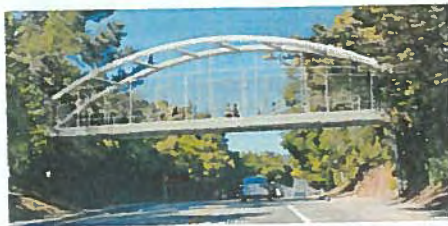
Option 4: Steel Tied Arch Bridge
