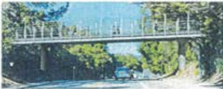
Option 1: Steel Girder Bridge
