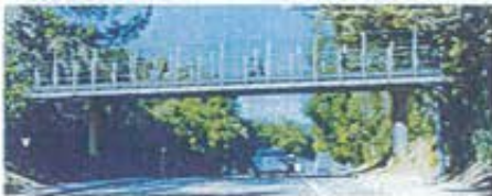
Option 1: Steel Girder Bridge
