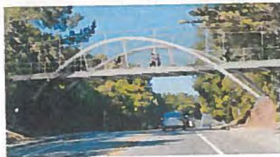
Option 5: Steel Inclined Arch Bridge
