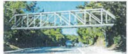
Option 3: Steel Howe Truss Bridge
