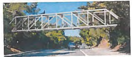
Option 3: Steel Howe Truss Bridge
