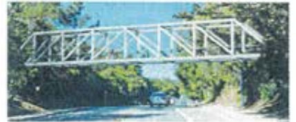
Option 3: Steel Howe Truss Bridge
