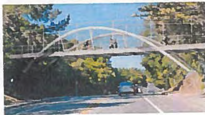
Option 5: Steel Inclined Arch Bridge
