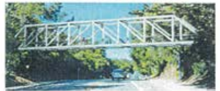
Option 3: Steel Howe Truss Bridge
