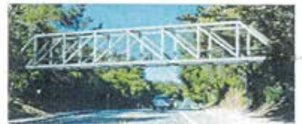
Option 3: Steel Howe Truss Bridge
