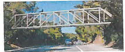
Option 3: Steel Howe Truss Bridge
