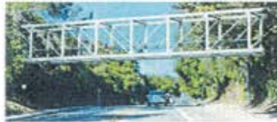
Option 2: Steel Pratt Truss Bridge
