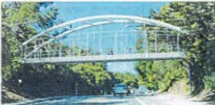
Option 4: Steel Tied Arch Bridge
