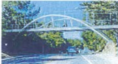
Option 5: Steel Inclined Arch Bridge
