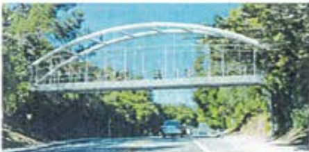
Option 4: Steel Tied Arch Bridge
