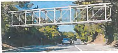
Option 2: Steel Pratt Truss Bridge
