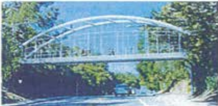
Option 4: Steel Tied Arch Bridge
