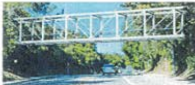
Option 2: Steel Pratt Truss Bridge
