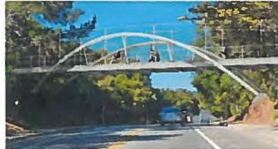
Option 5: Steel Inclined Arch Bridge
