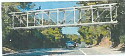
Option 2: Steel Pratt Truss Bridge
