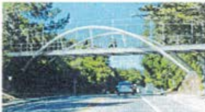
Option 5: Steel Inclined Arch Bridge
