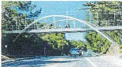
Option 5: Steel Inclined Arch Bridge
