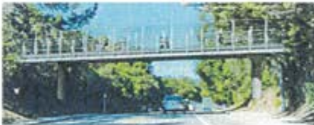
Option 1: Steel Girder Bridge
