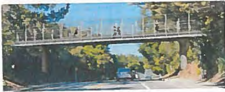
Option 1: Steel Girder Bridge
