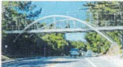
Option 5: Steel Inclined Arch Bridge
