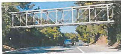
Option 2: Steel Pratt Truss Bridge
