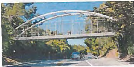
Option 4: Steel Tied Arch Bridge
