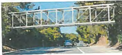
Option 2: Steel Pratt Truss Bridge
