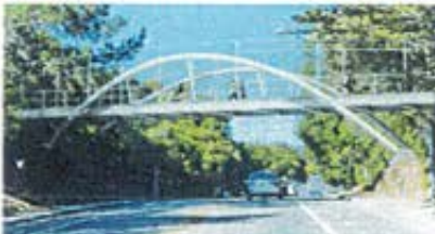
Option 5: Steel Inclined Arch Bridge
