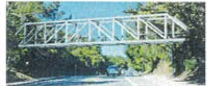
Option 3: Steel Howe Truss Bridge
