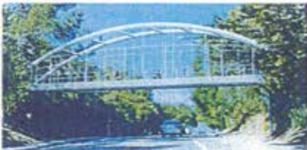
Option 4: Steel Tied Arch Bridge
