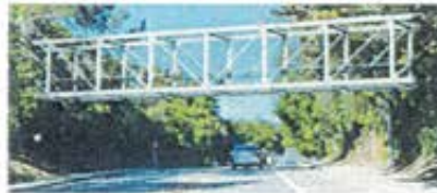
Option 2: Steel Pratt Truss Bridge
