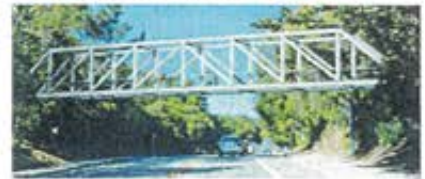
Option 3: Steel Howe Truss Bridge
