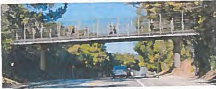
Option 1: Steel Girder Bridge
