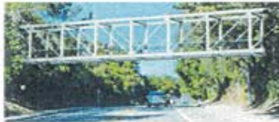
Option 2: Steel Pratt Truss Bridge
