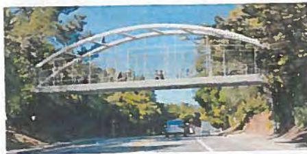
Option 4: Steel Tied Arch Bridge
