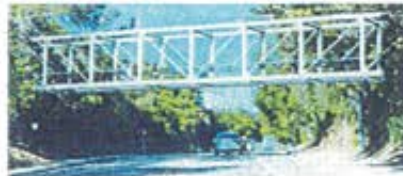
Option 2: Steel Pratt Truss Bridge
