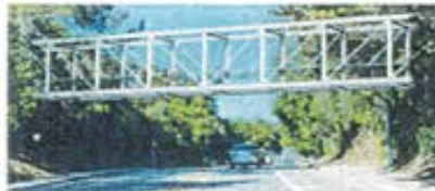
Option 2: Steel Pratt Truss Bridge
