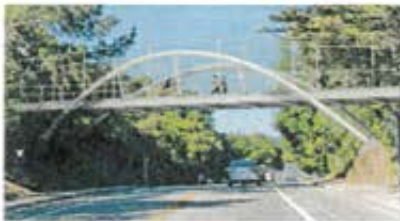
Option 5: Steel Inclined Arch Bridge
