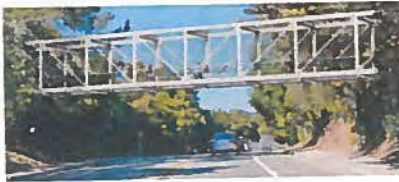
Option 2: Steel Pratt Truss Bridge
