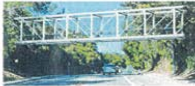
Option 2: Steel Pratt Truss Bridge
