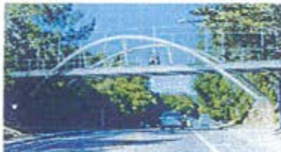
Option 5: Steel Inclined Arch Bridge
