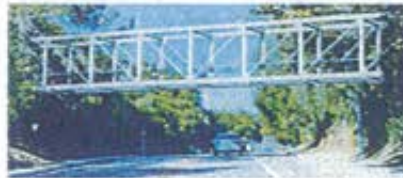
Option 2: Steel Pratt Truss Bridge
