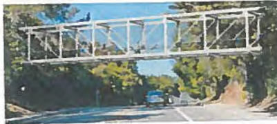
Option 2: Steel Pratt Truss Bridge
