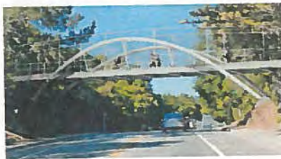
Option 5: Steel Inclined Arch Bridge
