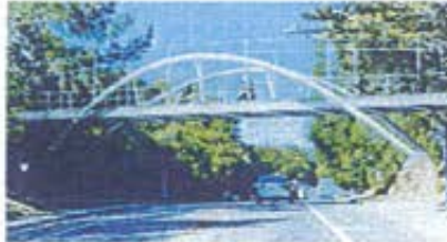
Option 5: Steel Inclined Arch Bridge
