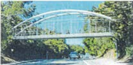
Option 4: Steel Tied Arch Bridge
