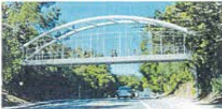
Option 4: Steel Tied Arch Bridge
