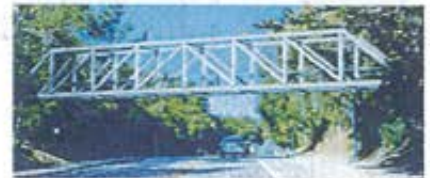
Option 3: Steel Howe Truss Bridge
