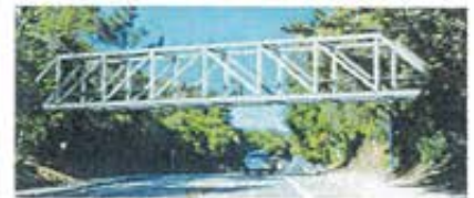
Option 3: Steel Howe Truss Bridge
