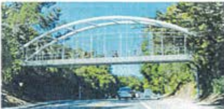
Option 4: Steel Tied Arch Bridge
