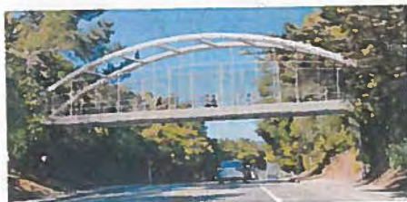
Option 4: Steel Tied Arch Bridge
