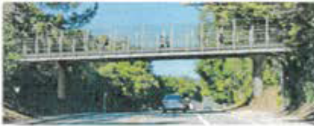
Option 1: Steel Girder Bridge
