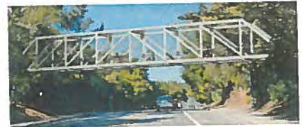
Option 3: Steel Howe Truss Bridge
