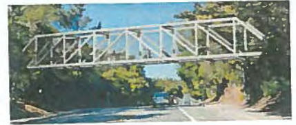
Option 3: Steel Howe Truss Bridge
