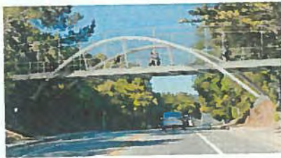
Option 5: Steel Inclined Arch Bridge
