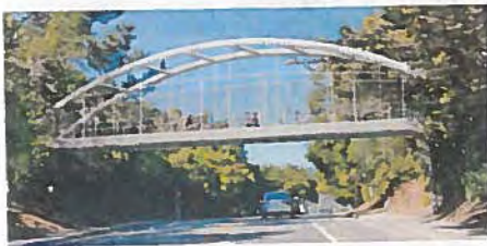
Option 4: Steel Tied Arch Bridge
