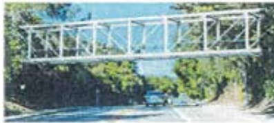
Option 2: Steel Pratt Truss Bridge
