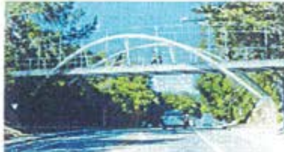
Option 5: Steel Inclined Arch Bridge
