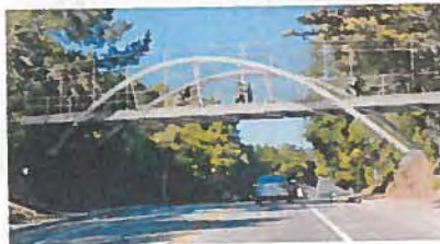
Option 5: Steel Inclined Arch Bridge
