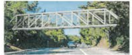
Option 3: Steel Howe Truss Bridge
