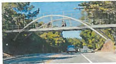
Option 5: Steel Inclined Arch Bridge
