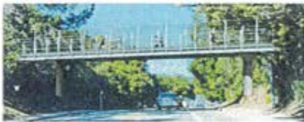
Option 1: Steel Girder Bridge
