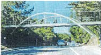
Option 5: Steel Inclined Arch Bridge
