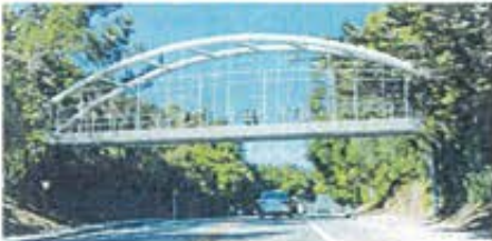
Option 4: Steel Tied Arch Bridge
