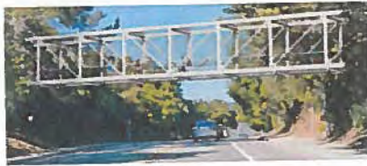
Option 2: Steel Pratt Truss Bridge
