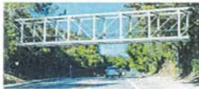
Option 2: Steel Pratt Truss Bridge
