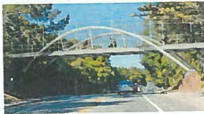
Option 5: Steel Inclined Arch Bridge
