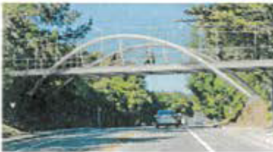
Option 5: Steel Inclined Arch Bridge
