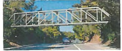
Option 3: Steel Howe Truss Bridge
