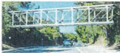
Option 2: Steel Pratt Truss Bridge
