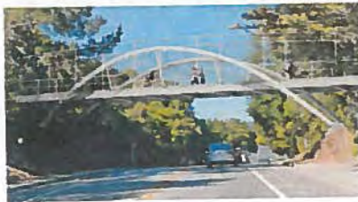
Option 5: Steel Inclined Arch Bridge
