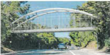
Option 4: Steel Tied Arch Bridge
