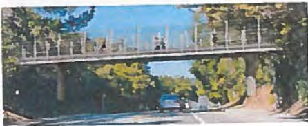
Option 1: Steel Girder Bridge
