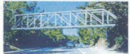
Option 3: Steel Howe Truss Bridge
