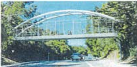
Option 4: Steel Tied Arch Bridge
