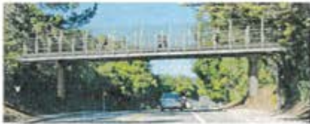
Option 1: Steel Girder Bridge
