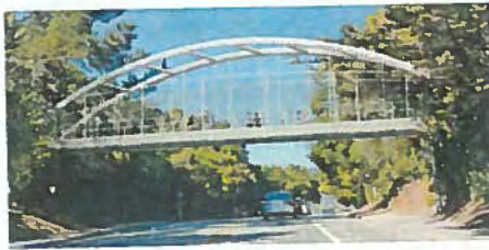
Option 4: Steel Tied Arch Bridge
