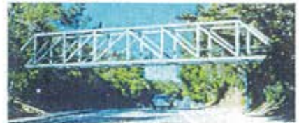
Option 3: Steel Howe Truss Bridge
