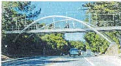
Option 5: Steel Inclined Arch Bridge
