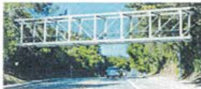
Option 2: Steel Pratt Truss Bridge
