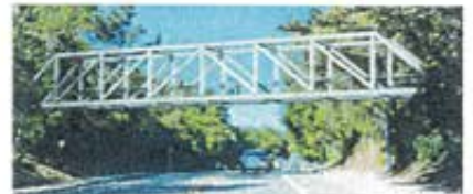
Option 3: Steel Howe Truss Bridge
