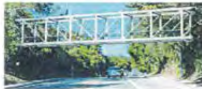
Option 2: Steel Pratt Truss Bridge
