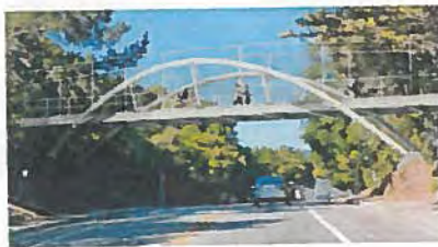
Option 5: Steel Inclined Arch Bridge
