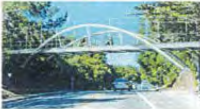
Option 5: Steel Inclined Arch Bridge
