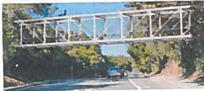
Option 2: Steel Pratt Truss Bridge
