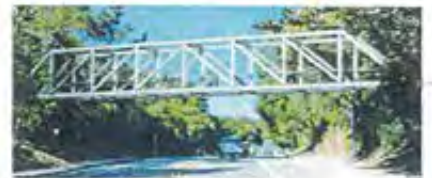
Option 3: Steel Howe Truss Bridge
