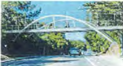
Option 5: Steel Inclined Arch Bridge
