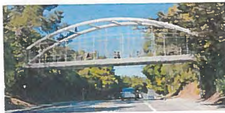
Option 4: Steel Tied Arch Bridge
