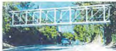
Option 2: Steel Pratt Truss Bridge
