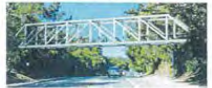
Option 3: Steel Howe Truss Bridge
