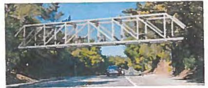
Option 3: Steel Howe Truss Bridge
