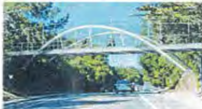
Option 5: Steel Inclined Arch Bridge
