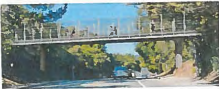
Option 1: Steel Girder Bridge
