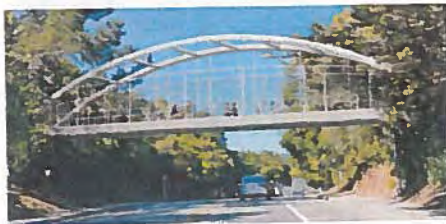
Option 4: Steel Tied Arch Bridge
