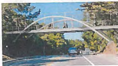
Option 5: Steel Inclined Arch Bridge
