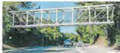
Option 2: Steel Pratt Truss Bridge
