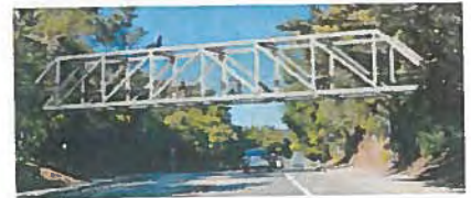
Option 3: Steel Howe Truss Bridge
