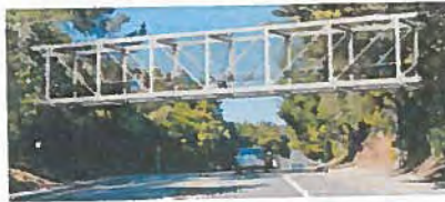
Option 2: Steel Pratt Truss Bridge
