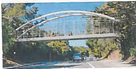
Option 4: Steel Tied Arch Bridge
