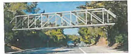
Option 3: Steel Howe Truss Bridge
