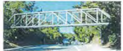
Option 3: Steel Howe Truss Bridge
