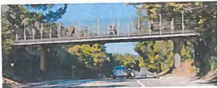
Option 1: Steel Girder Bridge
