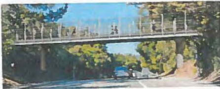
Option 1: Steel Girder Bridge
