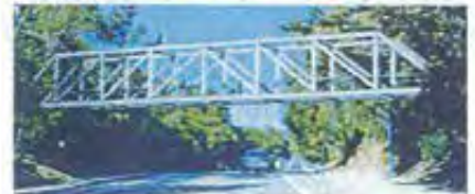
Option 3: Steel Howe Truss Bridge
