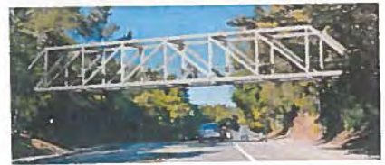
Option 3: Steel Howe Truss Bridge
