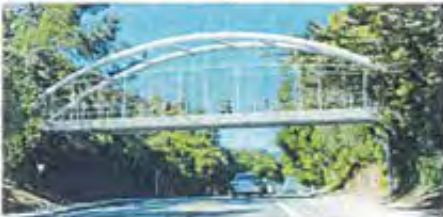
Option 4: Steel Tied Arch Bridge
