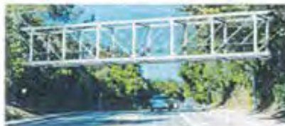
Option 2: Steel Pratt Truss Bridge
