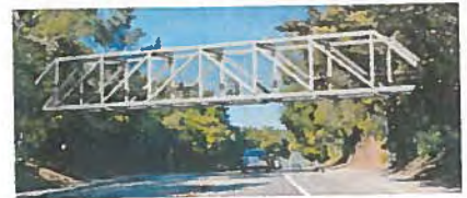
Option 3: Steel Howe Truss Bridge
