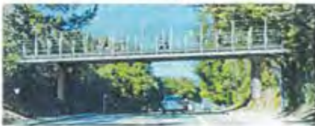
Option 1: Steel Girder Bridge
