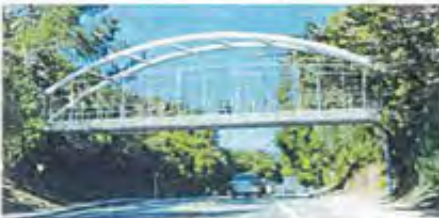
Option 4: Steel Tied Arch Bridge
