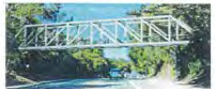
Option 3: Steel Howe Truss Bridge
