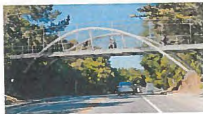
Option 5: Steel Inclined Arch Bridge
