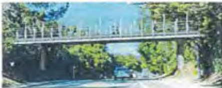
Option 1: Steel Girder Bridge
