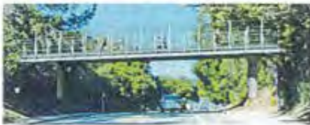
Option 1: Steel Girder Bridge
