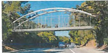
Option 4: Steel Tied Arch Bridge
