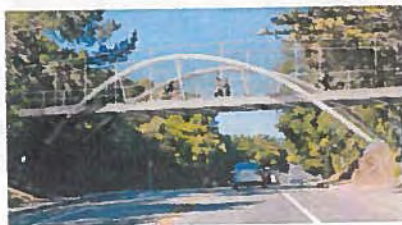
Option 5: Steel Inclined Arch Bridge
