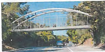
Option 4: Steel Tied Arch Bridge
