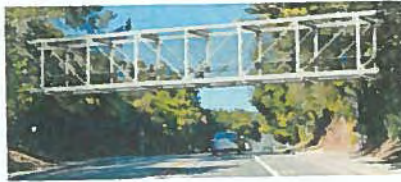
Option 2: Steel Pratt Truss Bridge
