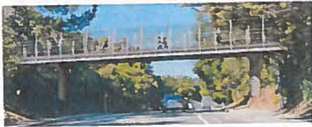
Option 1: Steel Girder Bridge
