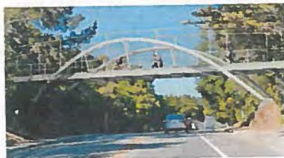
Option 5: Steel Inclined Arch Bridge
