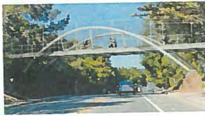
Option 5: Steel Inclined Arch Bridge
