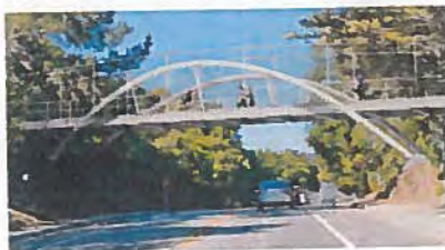
Option 5: Steel Inclined Arch Bridge
