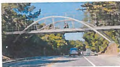
Option 5: Steel Inclined Arch Bridge
