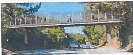
Option 1: Steel Girder Bridge
