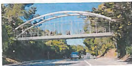
Option 4: Steel Tied Arch Bridge
