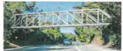
Option 3: Steel Howe Truss Bridge
