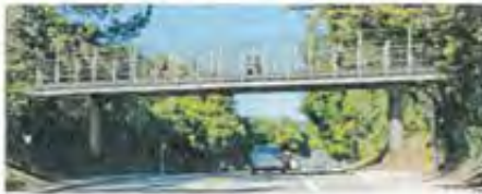
Option 1: Steel Girder Bridge
