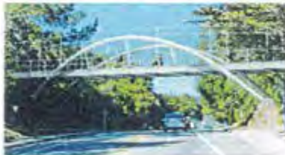
Option 5: Steel Inclined Arch Bridge
