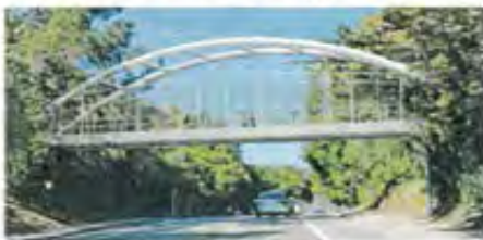
Option 4: Steel Tied Arch Bridge
