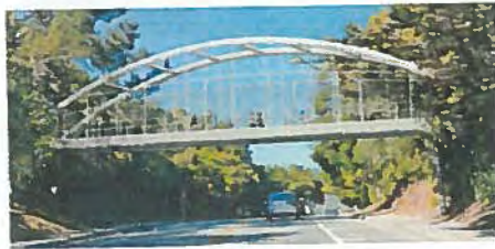
Option 4: Steel Tied Arch Bridge
