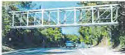
Option 2: Steel Pratt Truss Bridge
