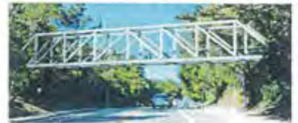
Option 3: Steel Howe Truss Bridge
