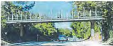
Option 1: Steel Girder Bridge
