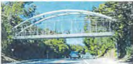
Option 4: Steel Tied Arch Bridge
