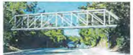
Option 3: Steel Howe Truss Bridge
