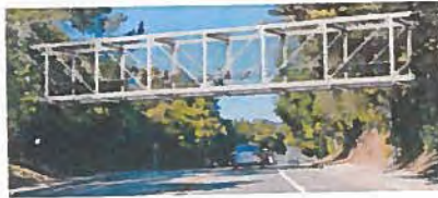
Option 2: Steel Pratt Truss Bridge
