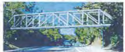
Option 3: Steel Howe Truss Bridge
