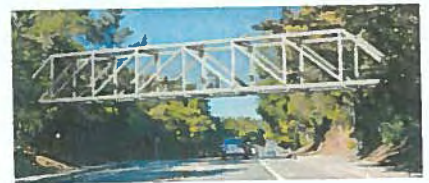
Option 3: Steel Howe Truss Bridge
