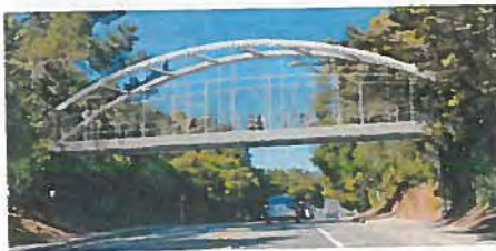
Option 4: Steel Tied Arch Bridge
