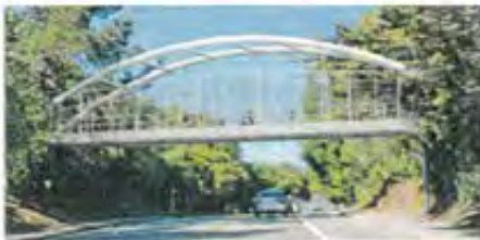
Option 4: Steel Tied Arch Bridge
