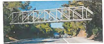
Option 3: Steel Howe Truss Bridge
