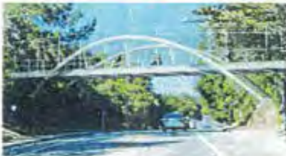
Option 5: Steel Inclined Arch Bridge
