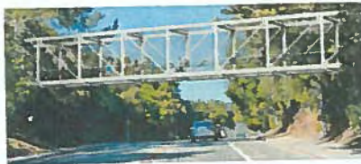
Option 2: Steel Pratt Truss Bridge
