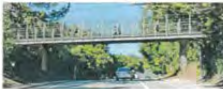
Option 1: Steel Girder Bridge
