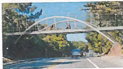
Option 5: Steel Inclined Arch Bridge
