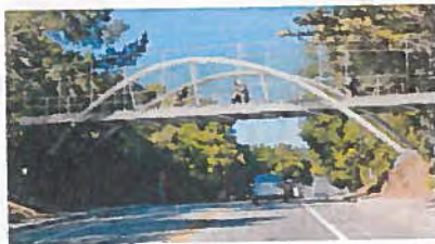
Option 5: Steel Inclined Arch Bridge
