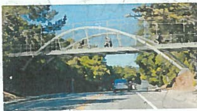
Option 5: Steel Inclined Arch Bridge
