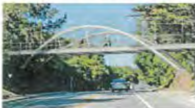
Option 5: Steel Inclined Arch Bridge
