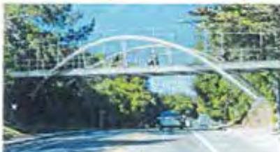
Option 5: Steel Inclined Arch Bridge
