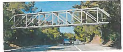
Option 3: Steel Howe Truss Bridge
