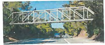
Option 3: Steel Howe Truss Bridge
