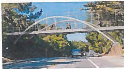
Option 5: Steel Inclined Arch Bridge
