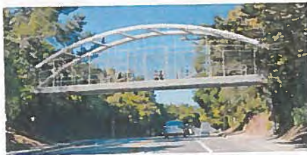
Option 4: Steel Tied Arch Bridge
