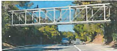
Option 2: Steel Pratt Truss Bridge
