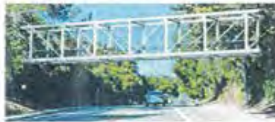
Option 2: Steel Pratt Truss Bridge
