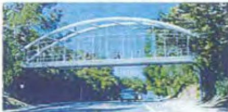
Option 4: Steel Tied Arch Bridge
