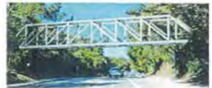
Option 3: Steel Howe Truss Bridge
