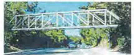
Option 3: Steel Howe Truss Bridge
