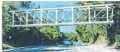
Option 2: Steel Pratt Truss Bridge
