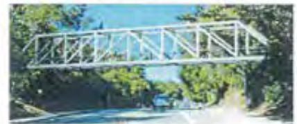
Option 3: Steel Howe Truss Bridge
