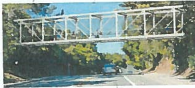
Option 2: Steel Pratt Truss Bridge
