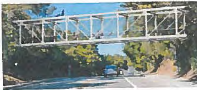
Option 2: Steel Pratt Truss Bridge
