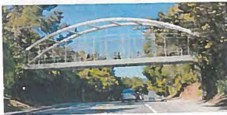
Option 4: Steel Tied Arch Bridge
