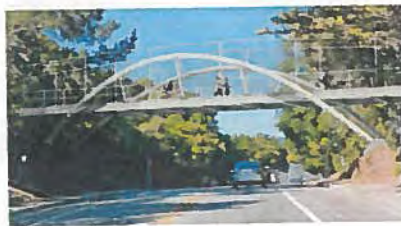
Option 5: Steel Inclined Arch Bridge
