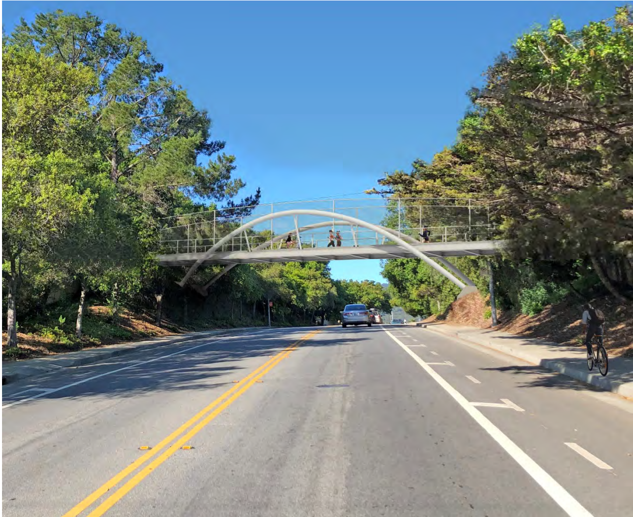
Figure 16. Rendering of a Steel Inclined Arch Bridge over Stevens Creek Boulevard. (Option 5)
