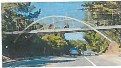
Option 5: Steel Inclined Arch Bridge
