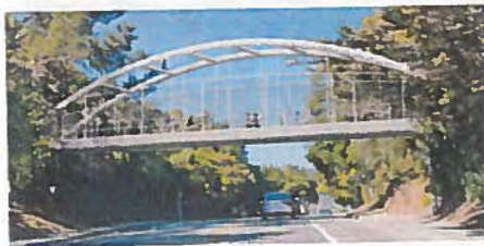
Option 4: Steel Tied Arch Bridge
