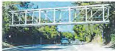
Option 2: Steel Pratt Truss Bridge
