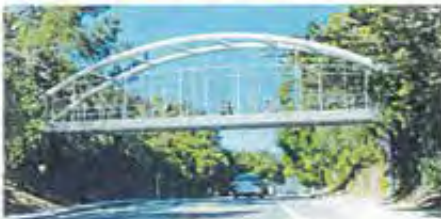
Option 4: Steel Tied Arch Bridge
