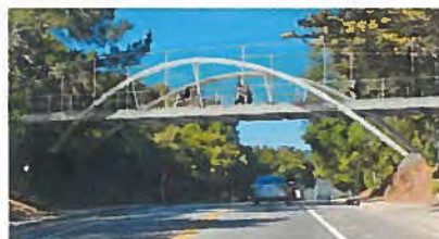
Option 5: Steel Inclined Arch Bridge
