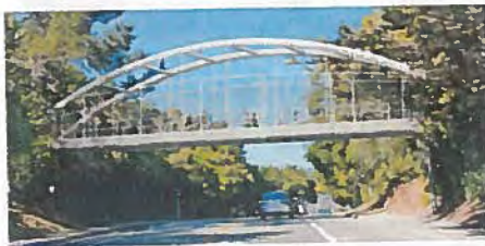
Option 4: Steel Tied Arch Bridge
