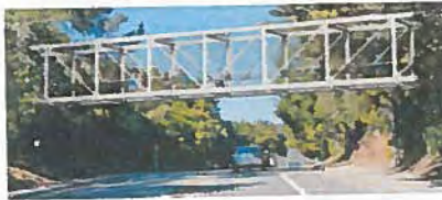
Option 2: Steel Pratt Truss Bridge
