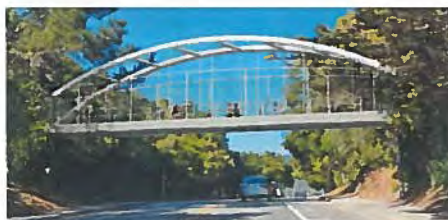
Option 4: Steel Tied Arch Bridge
