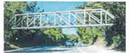
Option 3: Steel Howe Truss Bridge
