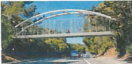
Option 4: Steel Tied Arch Bridge
