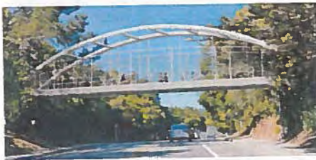
Option 4: Steel Tied Arch Bridge
