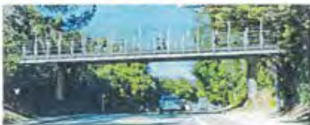
Option 1: Steel Girder Bridge
