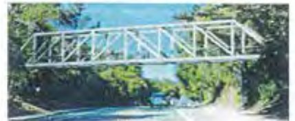
Option 3: Steel Howe Truss Bridge
