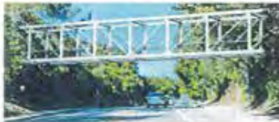
Option 2: Steel Pratt Truss Bridge
