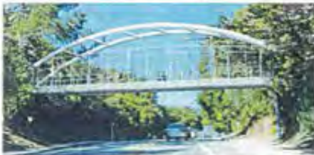
Option 4: Steel Tied Arch Bridge
