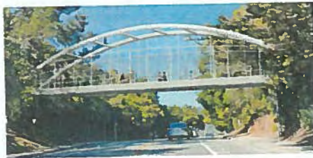
Option 4: Steel Tied Arch Bridge
