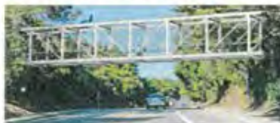
Option 2: Steel Pratt Truss Bridge
