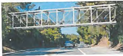
Option 2: Steel Pratt Truss Bridge
