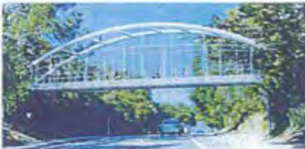
Option 4: Steel Tied Arch Bridge
