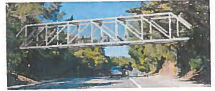
Option 3: Steel Howe Truss Bridge
