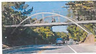
Option 5: Steel Inclined Arch Bridge
