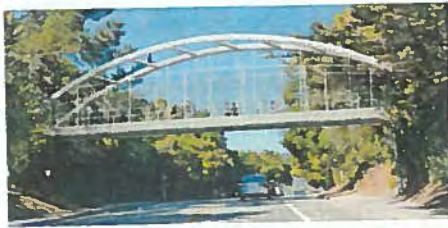
Option 4: Steel Tied Arch Bridge
