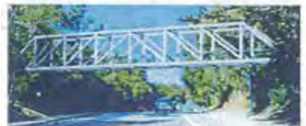
Option 3: Steel Howe Truss Bridge
