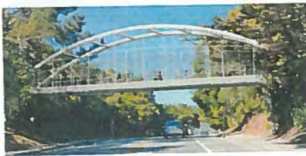
Option 4: Steel Tied Arch Bridge
