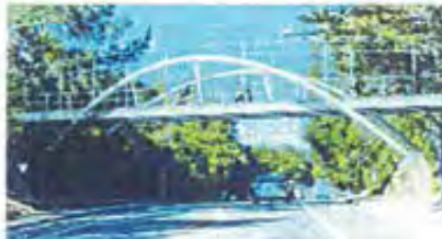
Option 5: Steel Inclined Arch Bridge
