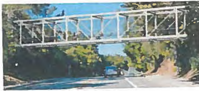
Option 2: Steel Pratt Truss Bridge
