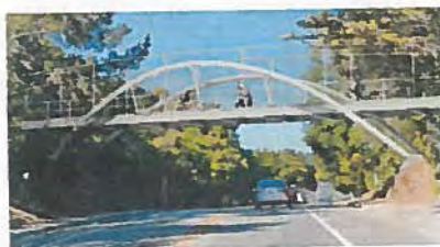
Option 5: Steel Inclined Arch Bridge
