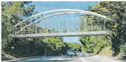
Option 4: Steel Tied Arch Bridge
