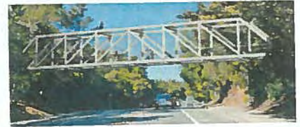
Option 3: Steel Howe Truss Bridge
