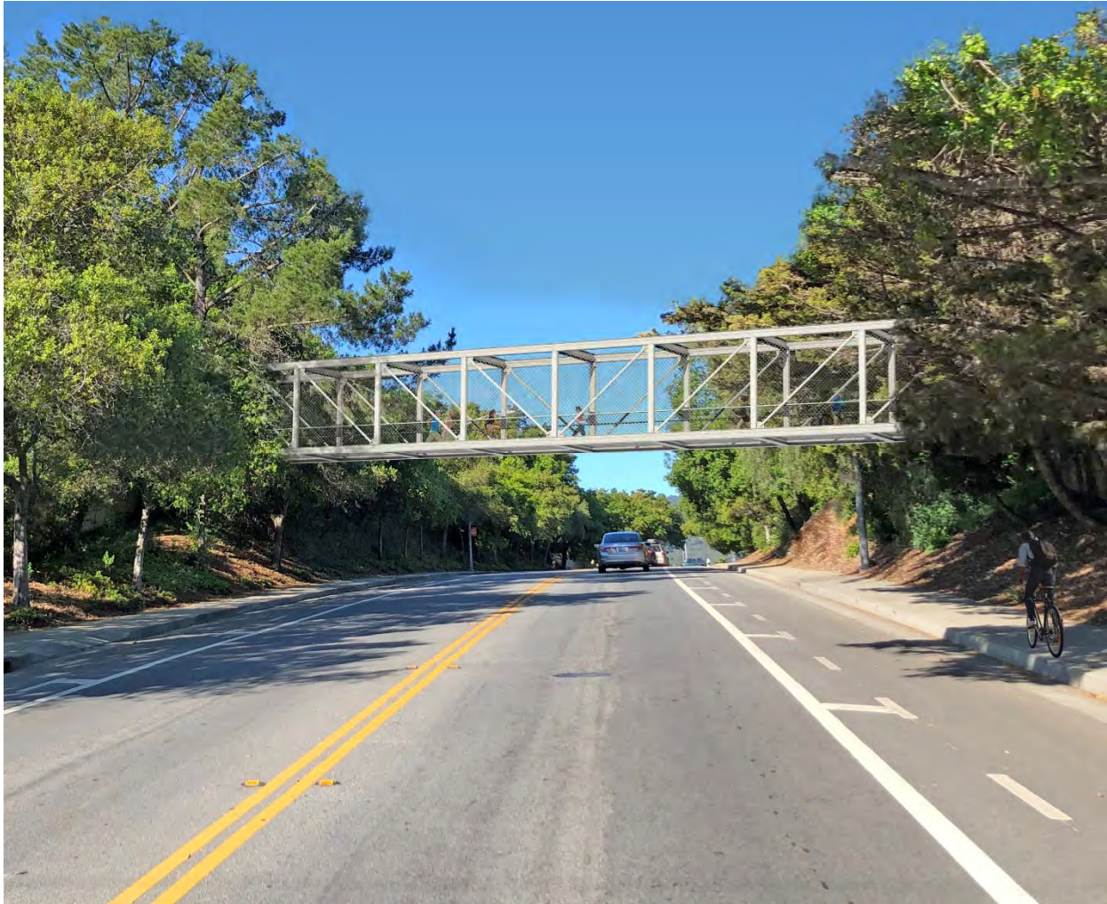
Figure 7. Rendering of a Steel Pratt Truss Bridge over Stevens Creek Boulevard. (Option 2)
