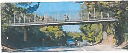
Option 1: Steel Girder Bridge
