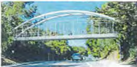
Option 4: Steel Tied Arch Bridge
