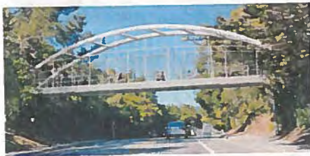
Option 4: Steel Tied Arch Bridge
