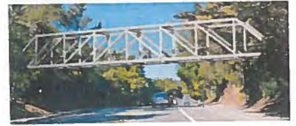
Option 3: Steel Howe Truss Bridge
