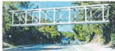
Option 2: Steel Pratt Truss Bridge
