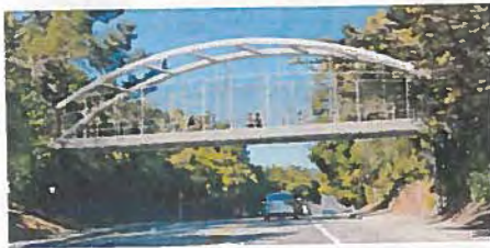
Option 4: Steel Tied Arch Bridge
