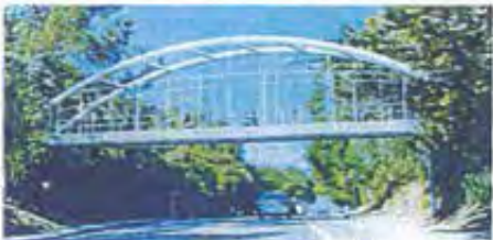
Option 4: Steel Tied Arch Bridge
