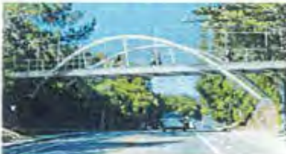
Option 5: Steel Inclined Arch Bridge
