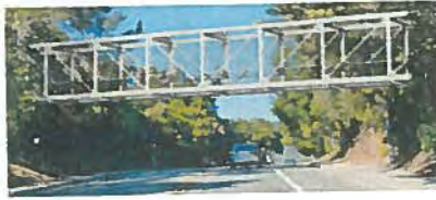
Option 2: Steel Pratt Truss Bridge
