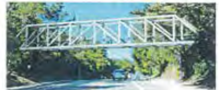
Option 3: Steel Howe Truss Bridge
