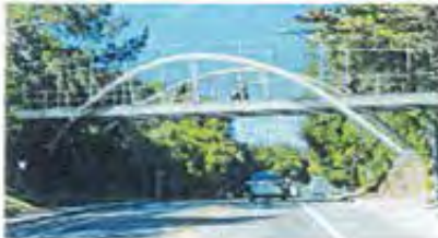
Option 5: Steel Inclined Arch Bridge
