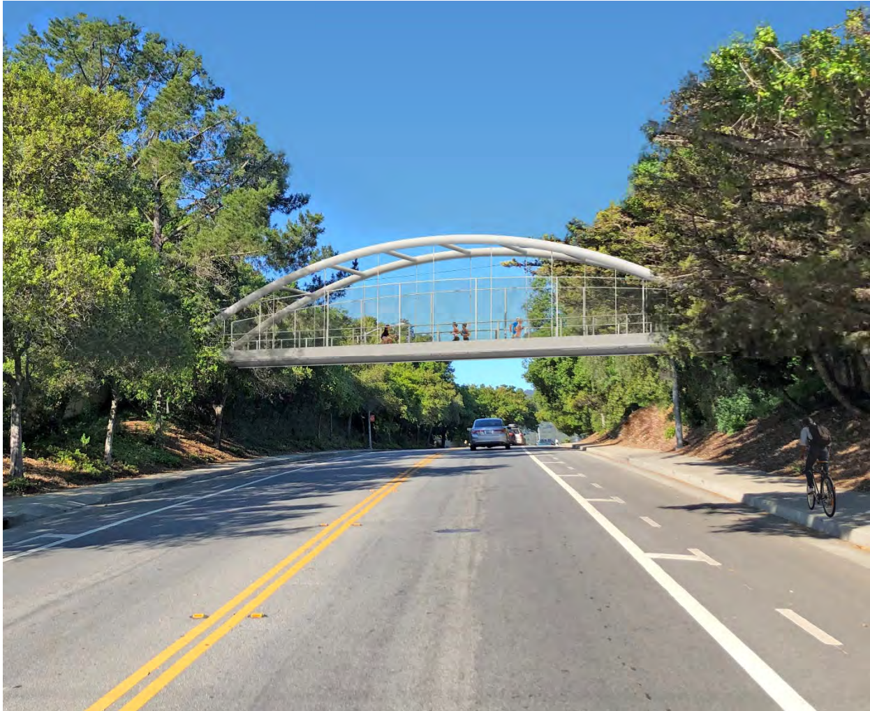
Figure 13. Rendering of a Steel Tied Arch Bridge over Stevens Creek Boulevard. (Option 4)
