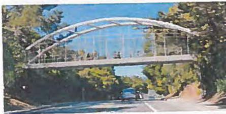
Option 4: Steel Tied Arch Bridge
