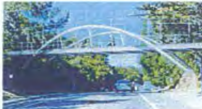
Option 5: Steel Inclined Arch Bridge
