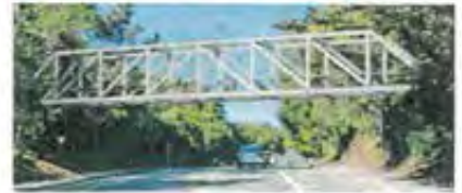
Option 3: Steel Howe Truss Bridge
