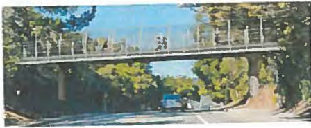
Option 1: Steel Girder Bridge
