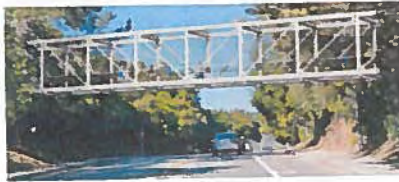
Option 2: Steel Pratt Truss Bridge
