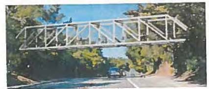
Option 3: Steel Howe Truss Bridge
