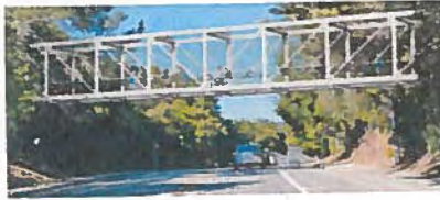
Option 2: Steel Pratt Truss Bridge
