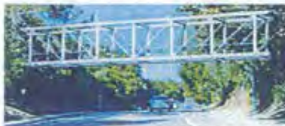
Option 2: Steel Pratt Truss Bridge
