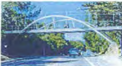
Option 5: Steel Inclined Arch Bridge
