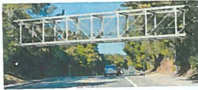
Option 2: Steel Pratt Truss Bridge
