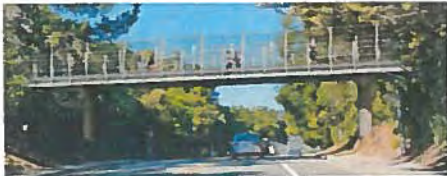
Option 1: Steel Girder Bridge
