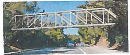
Option 3: Steel Howe Truss Bridge
