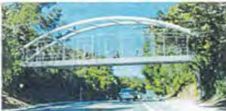
Option 4: Steel Tied Arch Bridge
