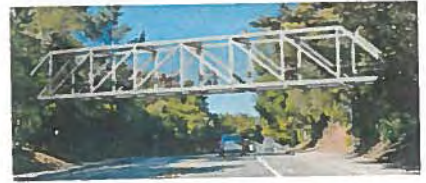
Option 3: Steel Howe Truss Bridge
