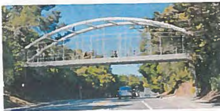
Option 4: Steel Tied Arch Bridge
