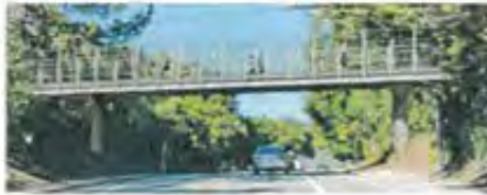
Option 1: Steel Girder Bridge
