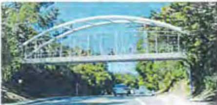
Option 4: Steel Tied Arch Bridge
