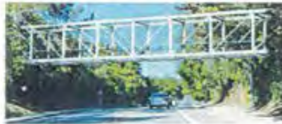
Option 2: Steel Pratt Truss Bridge
