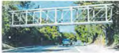
Option 2: Steel Pratt Truss Bridge
