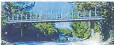
Option 1: Steel Girder Bridge
