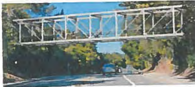
Option 2: Steel Pratt Truss Bridge
