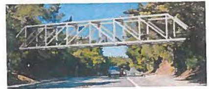
Option 3: Steel Howe Truss Bridge
