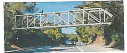
Option 3: Steel Howe Truss Bridge
