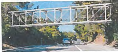
Option 2: Steel Pratt Truss Bridge
