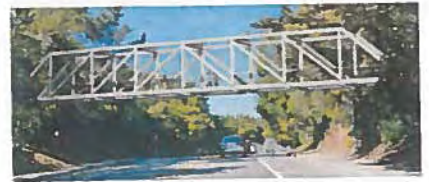
Option 3: Steel Howe Truss Bridge
