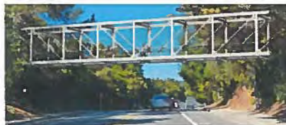
Option 2: Steel Pratt Truss Bridge
