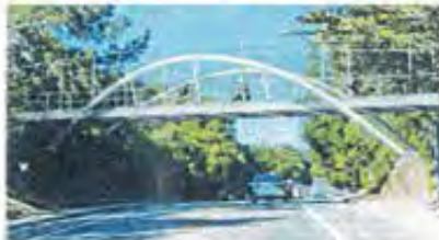
Option 5: Steel Inclined Arch Bridge
