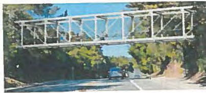
Option 2: Steel Pratt Truss Bridge
