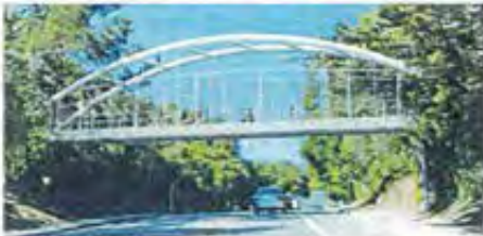
Option 4: Steel Tied Arch Bridge
