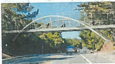
Option 5: Steel Inclined Arch Bridge
