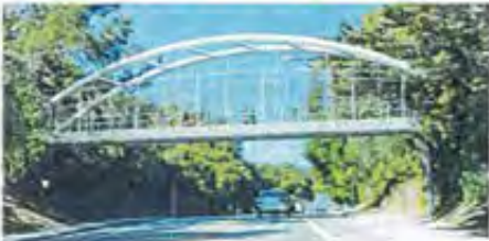
Option 4: Steel Tied Arch Bridge
