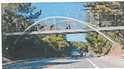
Option 5: Steel Inclined Arch Bridge
