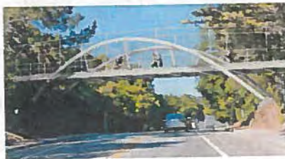
Option 5: Steel Inclined Arch Bridge
