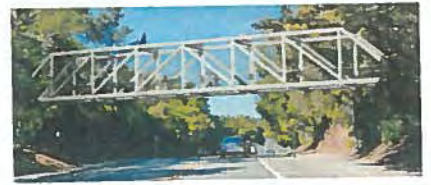
Option 3: Steel Howe Truss Bridge
