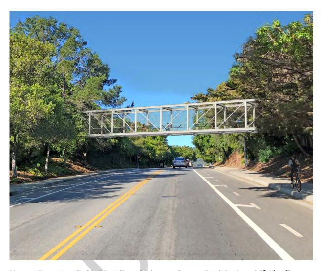
Figure 7. Rendering of a Steel Pratt Truss Bridge over Stevens Creek Boulevard. (Option 2)
