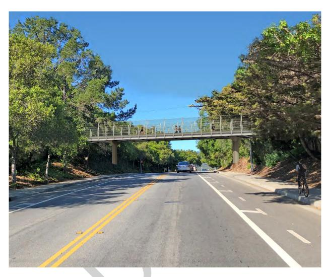
Figure 4. Rendering of a Steel Girder Bridge over Stevens Creek Boulevard. (Option 1)
