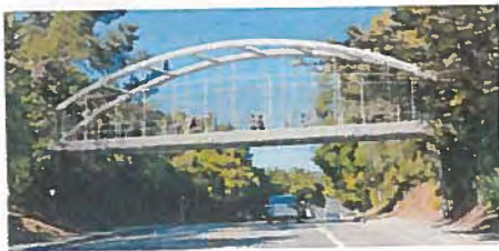
Option 4: Steel Tied Arch Bridge
