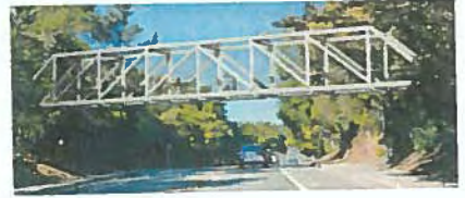
Option 3: Steel Howe Truss Bridge
