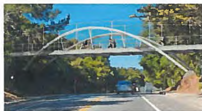
Option 5: Steel Inclined Arch Bridge
