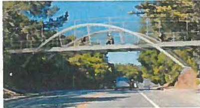
Option 5: Steel Inclined Arch Bridge
