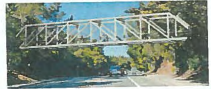
Option 3: Steel Howe Truss Bridge
