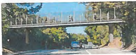
Option 1: Steel Girder Bridge
