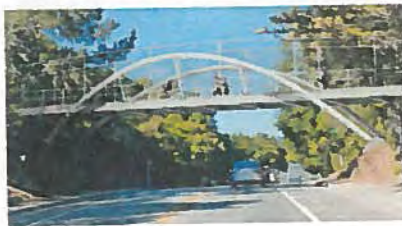
Option 5: Steel Inclined Arch Bridge
