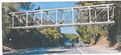
Option 2: Steel Pratt Truss Bridge
