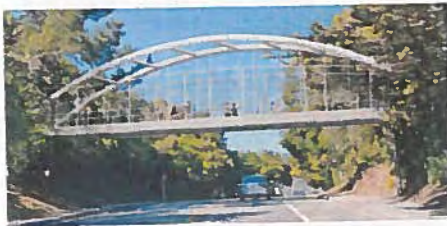
Option 4: Steel Tied Arch Bridge
