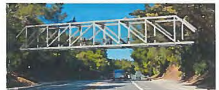
Option 3: Steel Howe Truss Bridge
