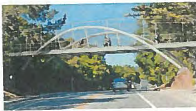
Option 5: Steel Inclined Arch Bridge
