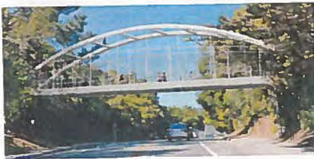
Option 4: Steel Tied Arch Bridge
