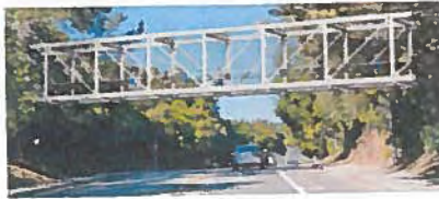
Option 2: Steel Pratt Truss Bridge
