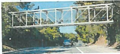
Option 2: Steel Pratt Truss Bridge
