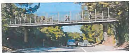
Option 1: Steel Girder Bridge
