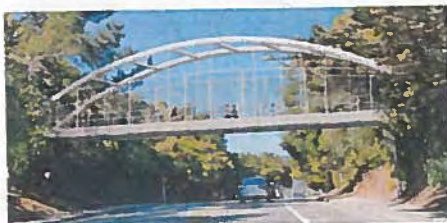
Option 4: Steel Tied Arch Bridge
