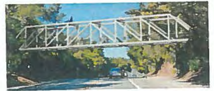
Option 3: Steel Howe Truss Bridge
