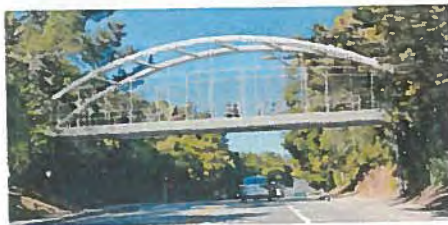
Option 4: Steel Tied Arch Bridge
