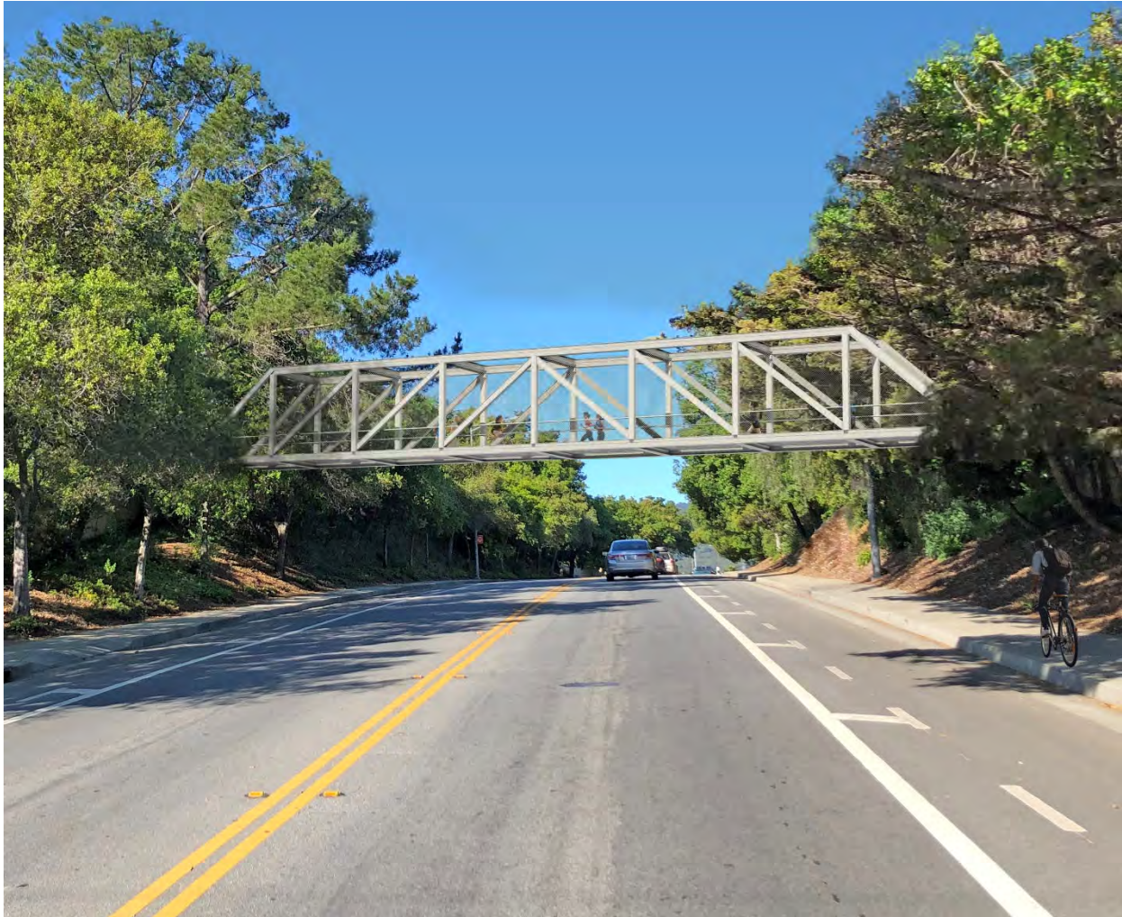
Figure 10. Rendering of a Steel Howe Truss Bridge over Stevens Creek Boulevard. (Option 3)
