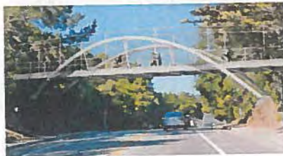
Option 5: Steel Inclined Arch Bridge
