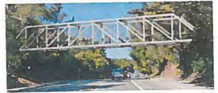
Option 3: Steel Howe Truss Bridge
