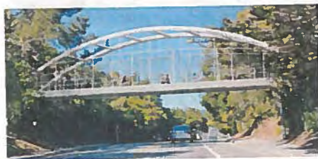
Option 4: Steel Tied Arch Bridge
