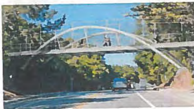
Option 5: Steel Inclined Arch Bridge
