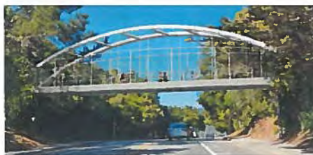
Option 4: Steel Tied Arch Bridge
