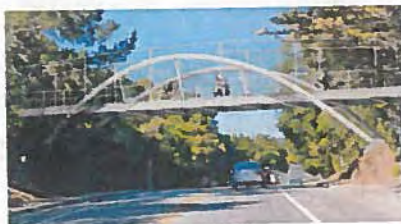
Option 5: Steel Inclined Arch Bridge
