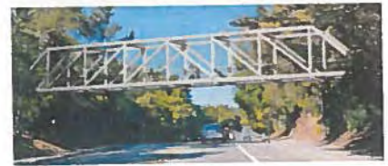
Option 3: Steel Howe Truss Bridge
