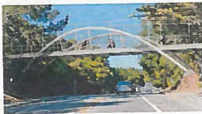
Option 5: Steel Inclined Arch Bridge
