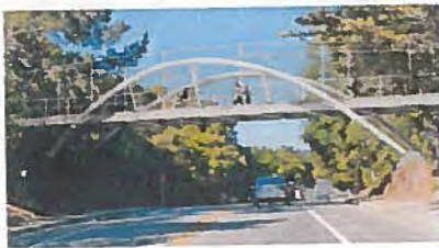
Option 5: Steel Inclined Arch Bridge
