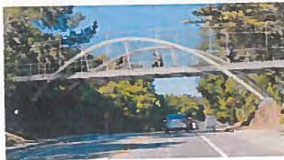
Option 5: Steel Inclined Arch Bridge
