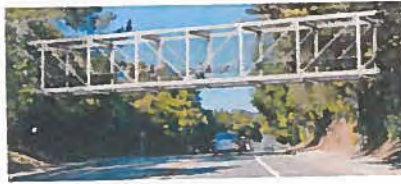
Option 2: Steel Pratt Truss Bridge
