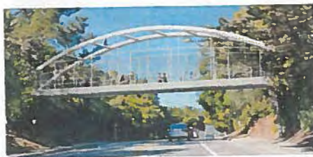
Option 4: Steel Tied Arch Bridge
