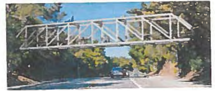
Option 3: Steel Howe Truss Bridge
