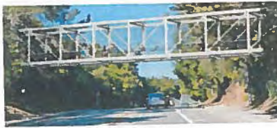
Option 2: Steel Pratt Truss Bridge
