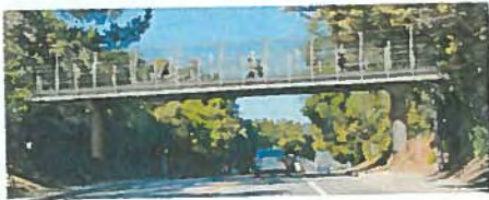
Option 1: Steel Girder Bridge
