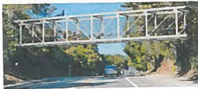
Option 2: Steel Pratt Truss Bridge
