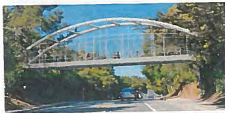
Option 4: Steel Tied Arch Bridge
