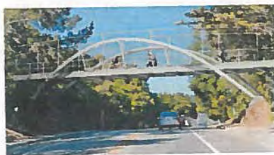
Option 5: Steel Inclined Arch Bridge
