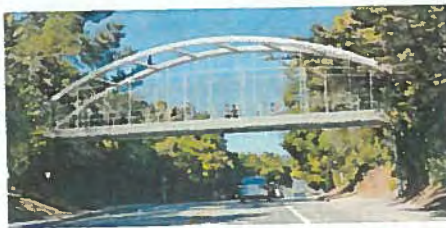
Option 4: Steel Tied Arch Bridge
