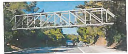
Option 3: Steel Howe Truss Bridge
