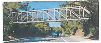
Option 3: Steel Howe Truss Bridge
