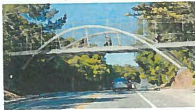
Option 5: Steel Inclined Arch Bridge
