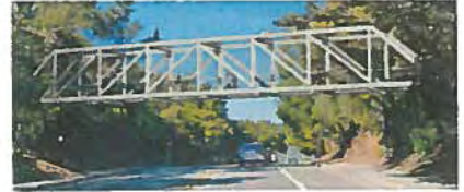
Option 3: Steel Howe Truss Bridge
