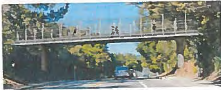
Option 1: Steel Girder Bridge
