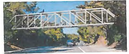
Option 3: Steel Howe Truss Bridge
