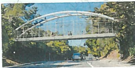
Option 4: Steel Tied Arch Bridge
