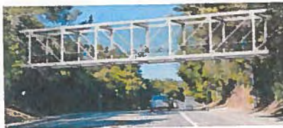
Option 2: Steel Pratt Truss Bridge
