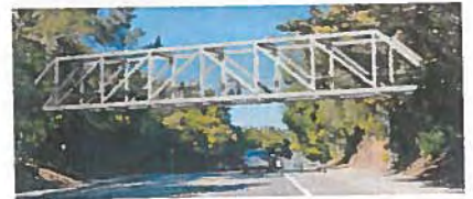
Option 3: Steel Howe Truss Bridge
