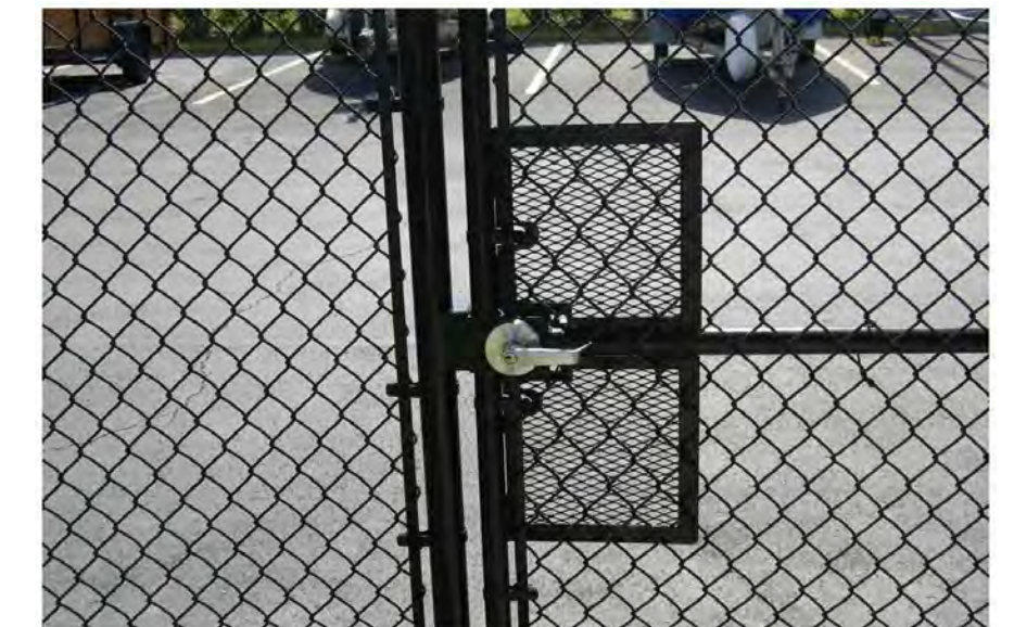
2 PEDESTRIAN GATE LOCK FROM THE INSIDE
