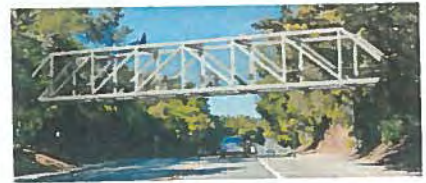
Option 3: Steel Howe Truss Bridge
