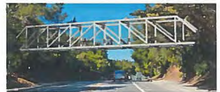
Option 3: Steel Howe Truss Bridge
