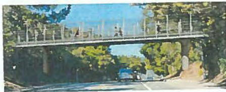
Option 1: Steel Girder Bridge
