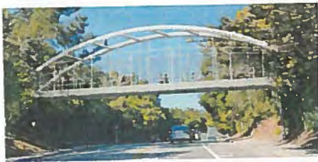
Option 4: Steel Tied Arch Bridge
