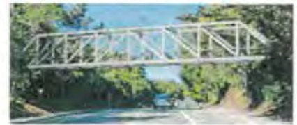
Option 3: Steel Howe Truss Bridge
