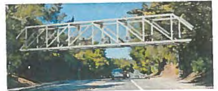
Option 3: Steel Howe Truss Bridge
