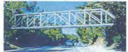
Option 3: Steel Howe Truss Bridge
