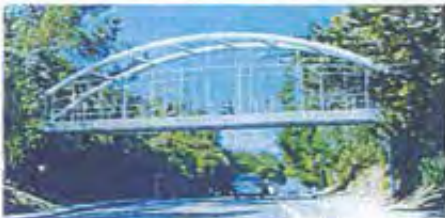
Option 4: Steel Tied Arch Bridge
