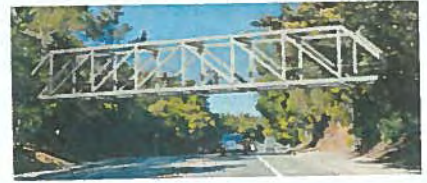
Option 3: Steel Howe Truss Bridge
