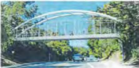
Option 4: Steel Tied Arch Bridge
