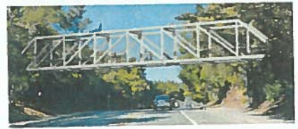
Option 3: Steel Howe Truss Bridge
