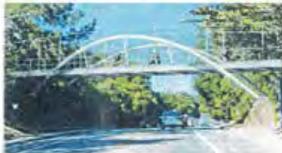
Option 5: Steel Inclined Arch Bridge
