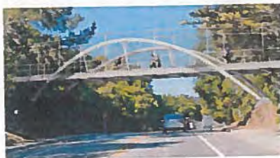
Option 5: Steel Inclined Arch Bridge
