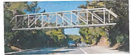
Option 3: Steel Howe Truss Bridge
