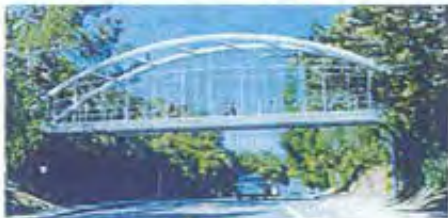
Option 4: Steel Tied Arch Bridge
