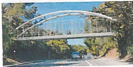
Option 4: Steel Tied Arch Bridge
