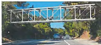
Option 2: Steel Pratt Truss Bridge
