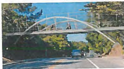
Option 5: Steel Inclined Arch Bridge
