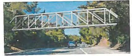
Option 3: Steel Howe Truss Bridge
