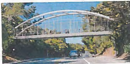
Option 4: Steel Tied Arch Bridge
