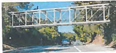
Option 2: Steel Pratt Truss Bridge
