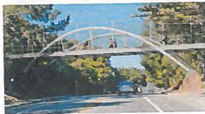
Option 5: Steel Inclined Arch Bridge
