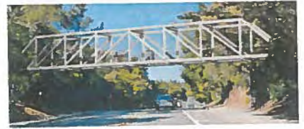
Option 3: Steel Howe Truss Bridge
