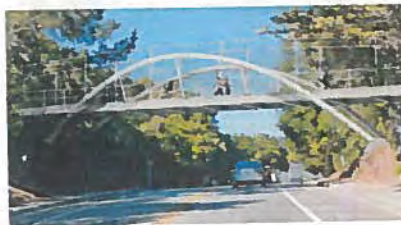
Option 5: Steel Inclined Arch Bridge
