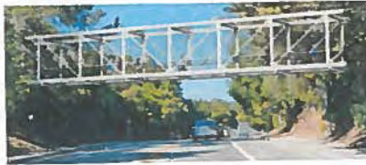
Option 2: Steel Pratt Truss Bridge
