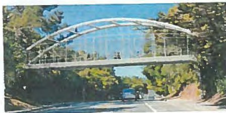
Option 4: Steel Tied Arch Bridge
