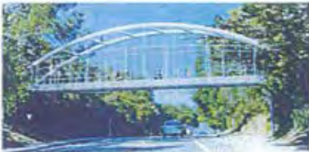
Option 4: Steel Tied Arch Bridge
