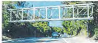
Option 2: Steel Pratt Truss Bridge
