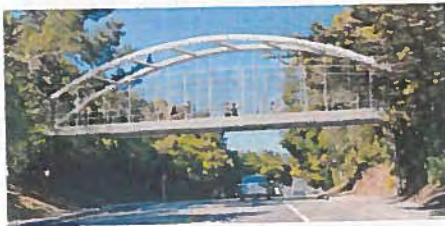
Option 4: Steel Tied Arch Bridge
