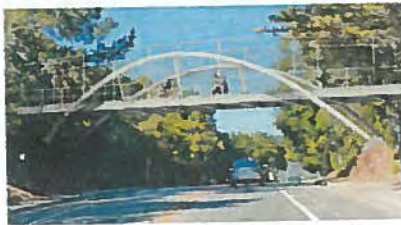
Option 5: Steel Inclined Arch Bridge
