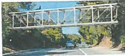
Option 2: Steel Pratt Truss Bridge
