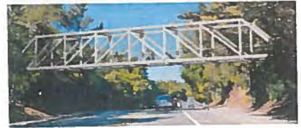
Option 3: Steel Howe Truss Bridge
