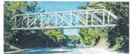
Option 3: Steel Howe Truss Bridge
