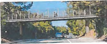
Option 1: Steel Girder Bridge
