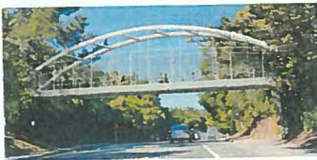
Option 4: Steel Tied Arch Bridge
