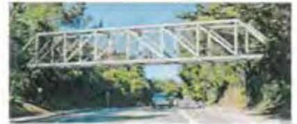
Option 3: Steel Howe Truss Bridge
