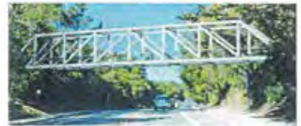
Option 3: Steel Howe Truss Bridge
