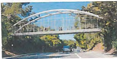
Option 4: Steel Tied Arch Bridge
