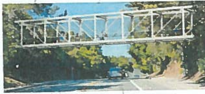
Option 2: Steel Pratt Truss Bridge
