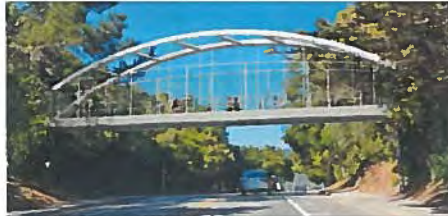
Option 4: Steel Tied Arch Bridge
