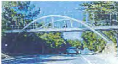
Option 5: Steel Inclined Arch Bridge
