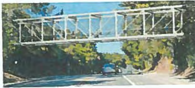
Option 2: Steel Pratt Truss Bridge
