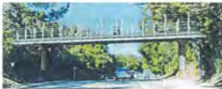
Option 1: Steel Girder Bridge
