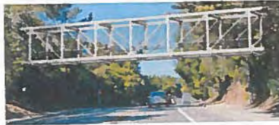
Option 2: Steel Pratt Truss Bridge
