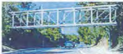
Option 2: Steel Pratt Truss Bridge
