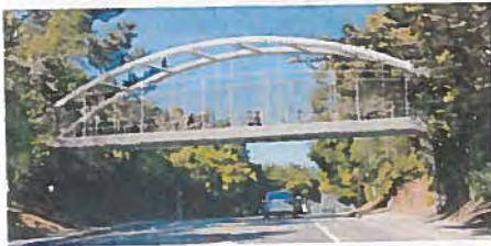
Option 4: Steel Tied Arch Bridge
