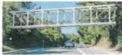
Option 2: Steel Pratt Truss Bridge
