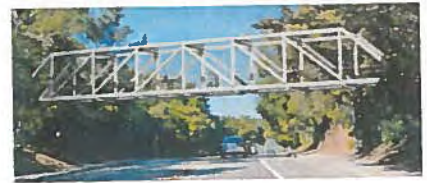
Option 3: Steel Howe Truss Bridge
