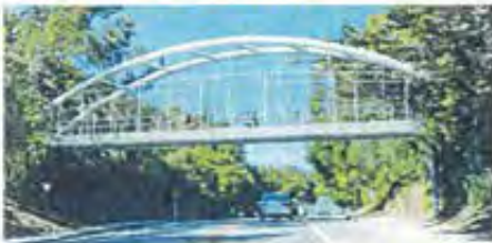
Option 4: Steel Tied Arch Bridge
