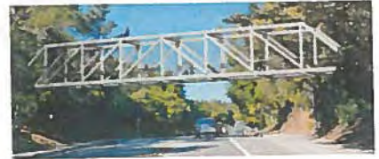
Option 3: Steel Howe Truss Bridge
