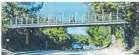
Option 1: Steel Girder Bridge
