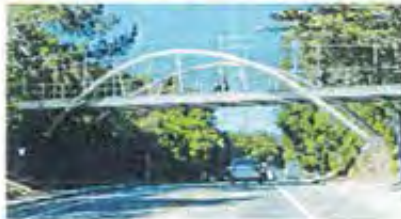
Option 5: Steel Inclined Arch Bridge
