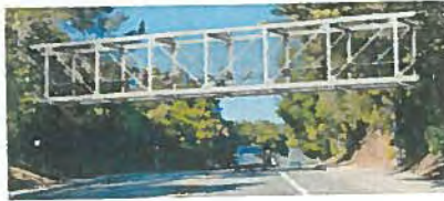
Option 2: Steel Pratt Truss Bridge
