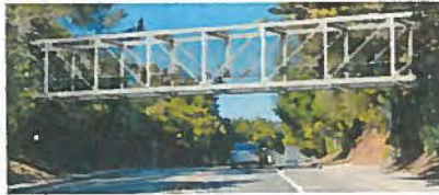
Option 2: Steel Pratt Truss Bridge
