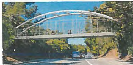
Option 4: Steel Tied Arch Bridge
