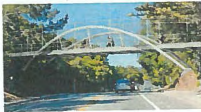
Option 5: Steel Inclined Arch Bridge
