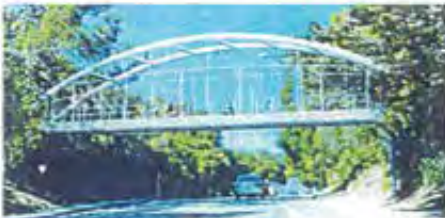
Option 4: Steel Tied Arch Bridge
