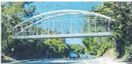
Option 4: Steel Tied Arch Bridge
