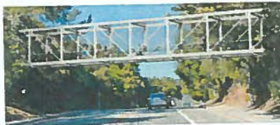
Option 2: Steel Pratt Truss Bridge
