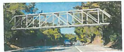
Option 3: Steel Howe Truss Bridge
