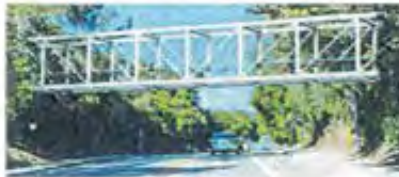
Option 2: Steel Pratt Truss Bridge
