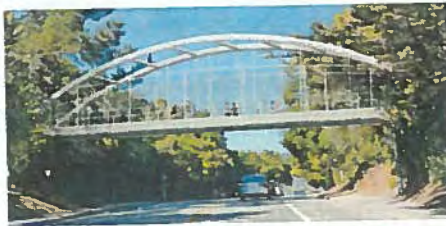
Option 4: Steel Tied Arch Bridge
