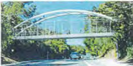
Option 4: Steel Tied Arch Bridge
