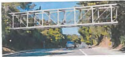
Option 2: Steel Pratt Truss Bridge
