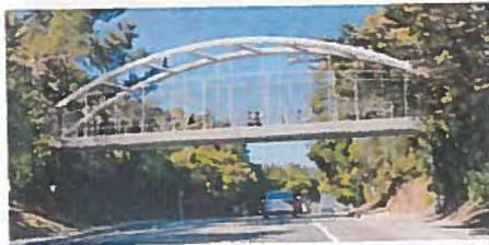
Option 4: Steel Tied Arch Bridge
