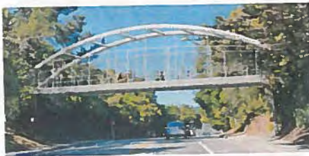
Option 4: Steel Tied Arch Bridge
