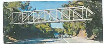
Option 3: Steel Howe Truss Bridge
