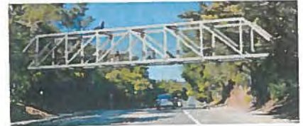
Option 3: Steel Howe Truss Bridge
