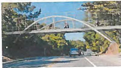
Option 5: Steel Inclined Arch Bridge
