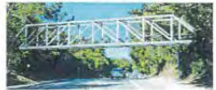
Option 3: Steel Howe Truss Bridge
