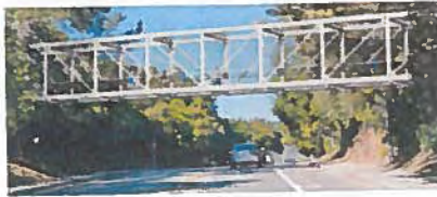
Option 2: Steel Pratt Truss Bridge
