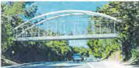
Option 4: Steel Tied Arch Bridge
