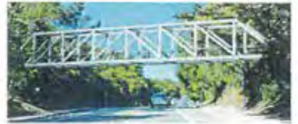
Option 3: Steel Howe Truss Bridge
