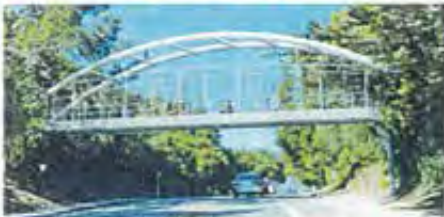
Option 4: Steel Tied Arch Bridge
