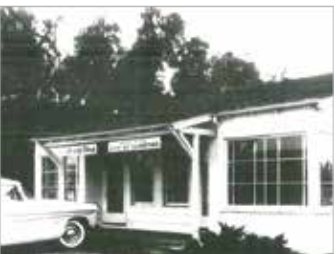
Interim City Hall 10321 South De Anza Boulevard
