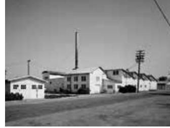
Woelffel Cannery 10120 Imperial Avenue Demolished
