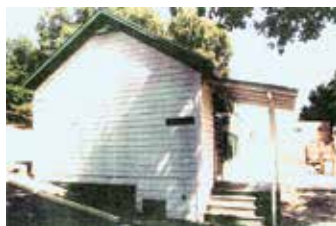
Montebello School 15101 Montebello Road
