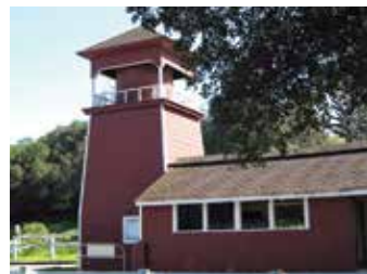
Enoch J. Parrish Tank House 22221 McClellan Road McClellan Ranch Park
