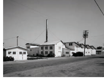
Woelffel Cannery 10120 Imperial Avenue Demolished
