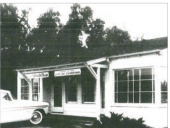
Interim City Hall 10321 South De Anza Boulevard
