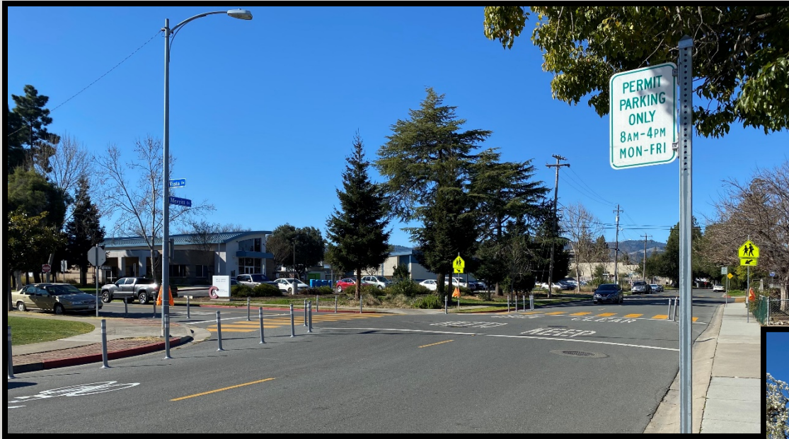
Pilot Bulb-Outs at Vista & Merritt, near Lawson Middle School
