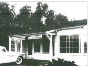
Interim City Hall 10321 South De Anza Boulevard
