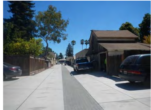
Figure 2-5 Infiltration trench, San Jose (Source: City of San Jose)
