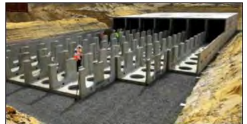
Figure 2-9 Subsurface vault, under construction (Source: Conteches.com)
