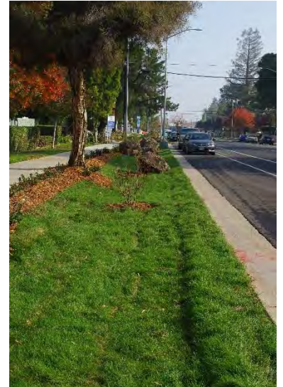
Figure 2-2 Stormwater planter, Hacienda Avenue, Campbell (Source: City of Campbell)
