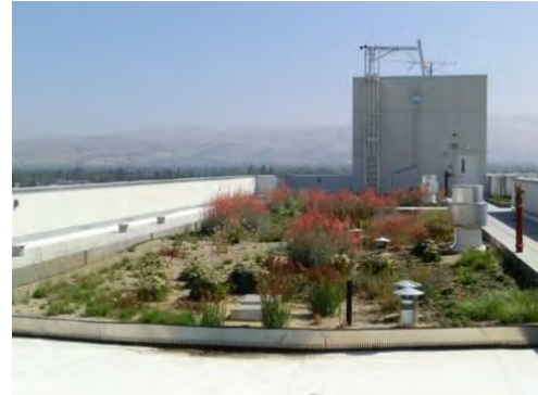
Figure 2-7 Green roof at Fourth Street Apartments, San José (Source: EOA)
