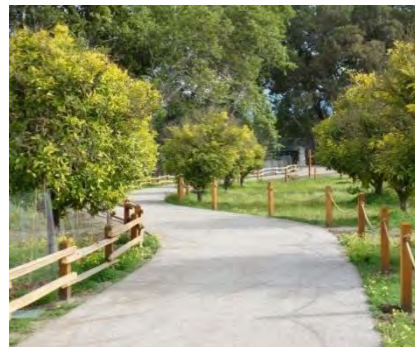
Figure 2-11 Pervious concrete bike path and walkway at Blackberry Farm. (Source: City of Cupertino)
