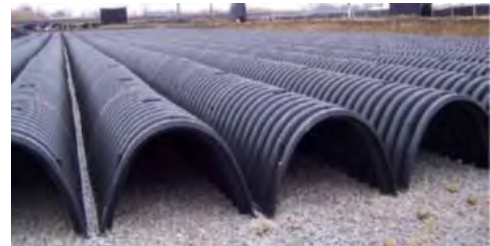
Figure 2-6 Subsurface infiltration system (Source: Conteches.com)
