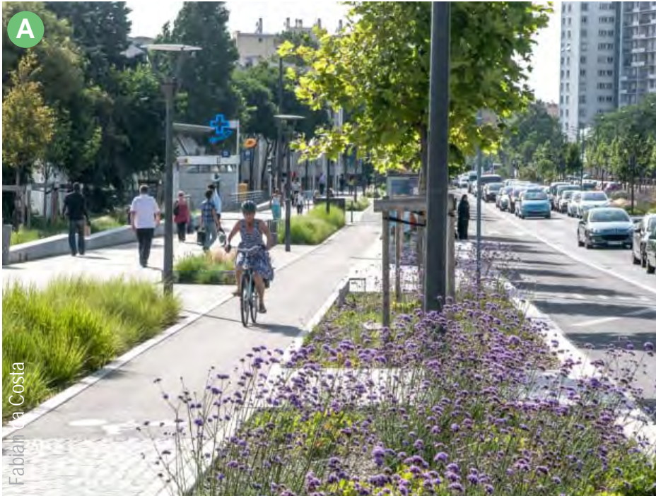
Example of Integration of Bioretention with Bike and Pedestrian Crossings in Lyon, France
