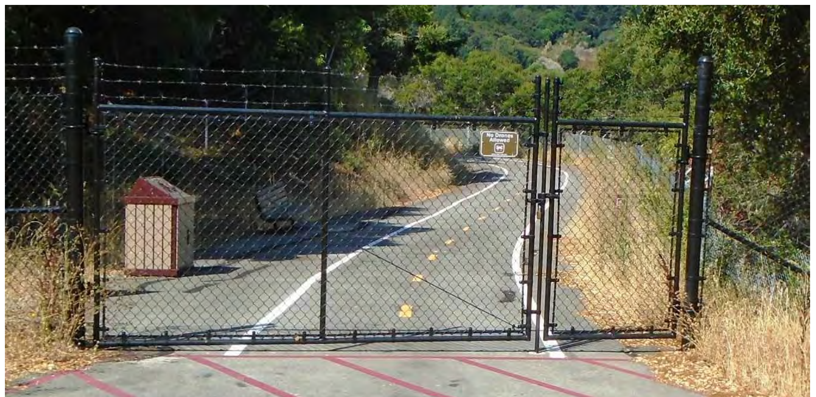
1 TRAIL ENTRY GATE "CRYSTAL SPRINGS RESERVOIR" TYPE
