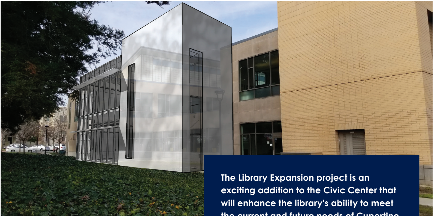
View of the southeast facade (ehdd)
