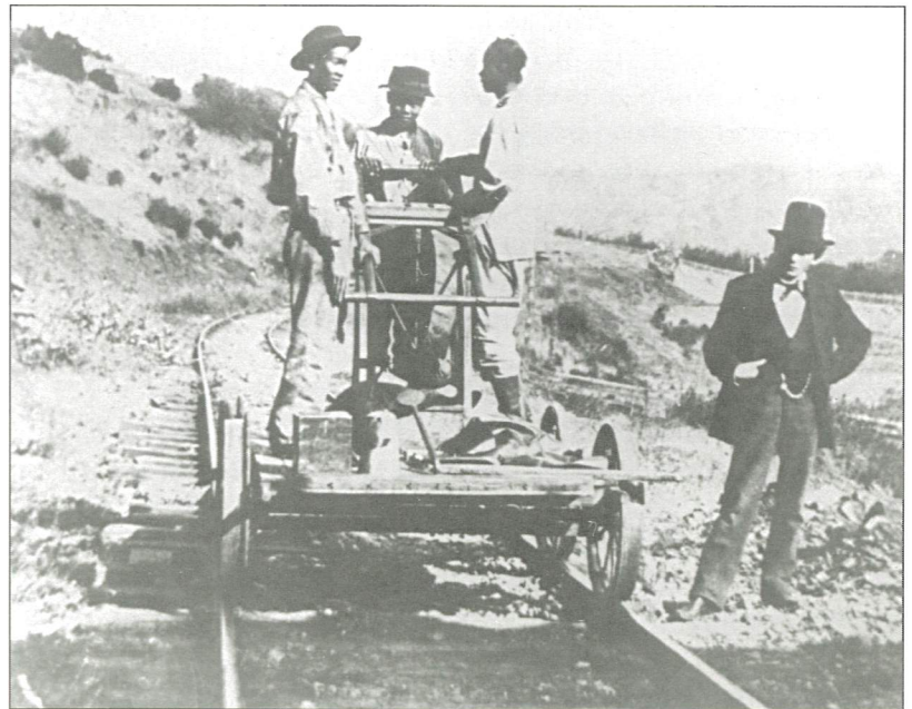
Chinese working on the California Railroad, ca 1860s.
