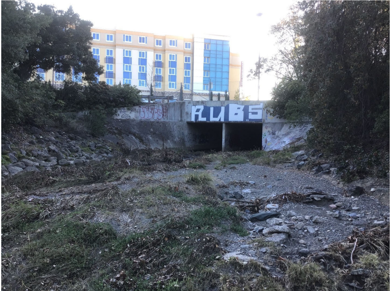
Photo 7. Box culvert where Calabazas Creek enters the project area.
