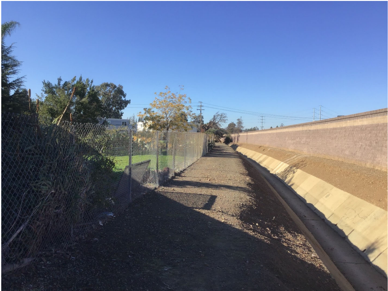
Photo 1. Developed land cover within the project area. Junipero Serra Channel with hardpack access road, chain link fence, and sound wall.
