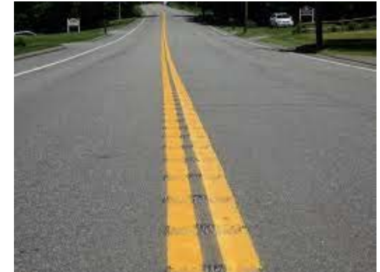
Install centerline rumble strips
