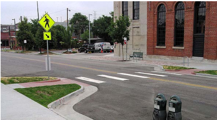
Install/upgrade pedestrian crossing (with enhanced safety features)
