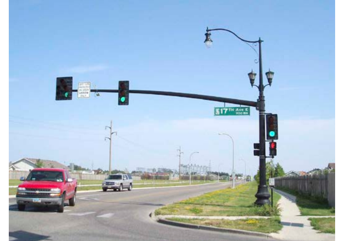
Convert signal to mast arm
