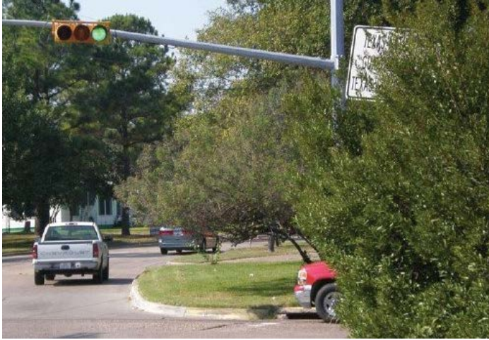
Improve sight distance
