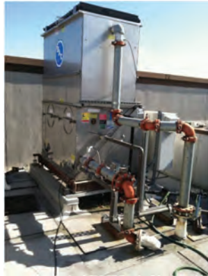
Figure 5A (Closed-Circuit 70 Ton Cooling Tower)
