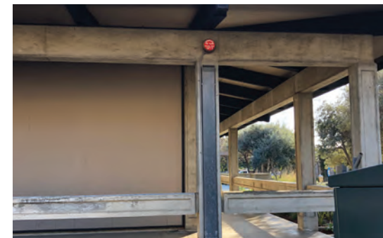
Typical Exterior Structure at Main Level
