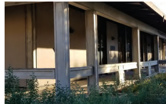
Typical Concrete Columns and Handrails at Porch Area
