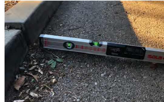
More than 7% Grade
