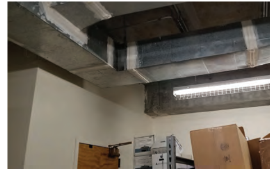
Deteriorated Ductwork
