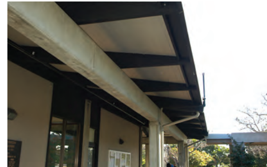
Typical Exterior Beam and Soffit Condition
