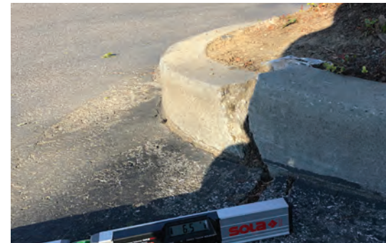
Sidewalk/Paving Crack
