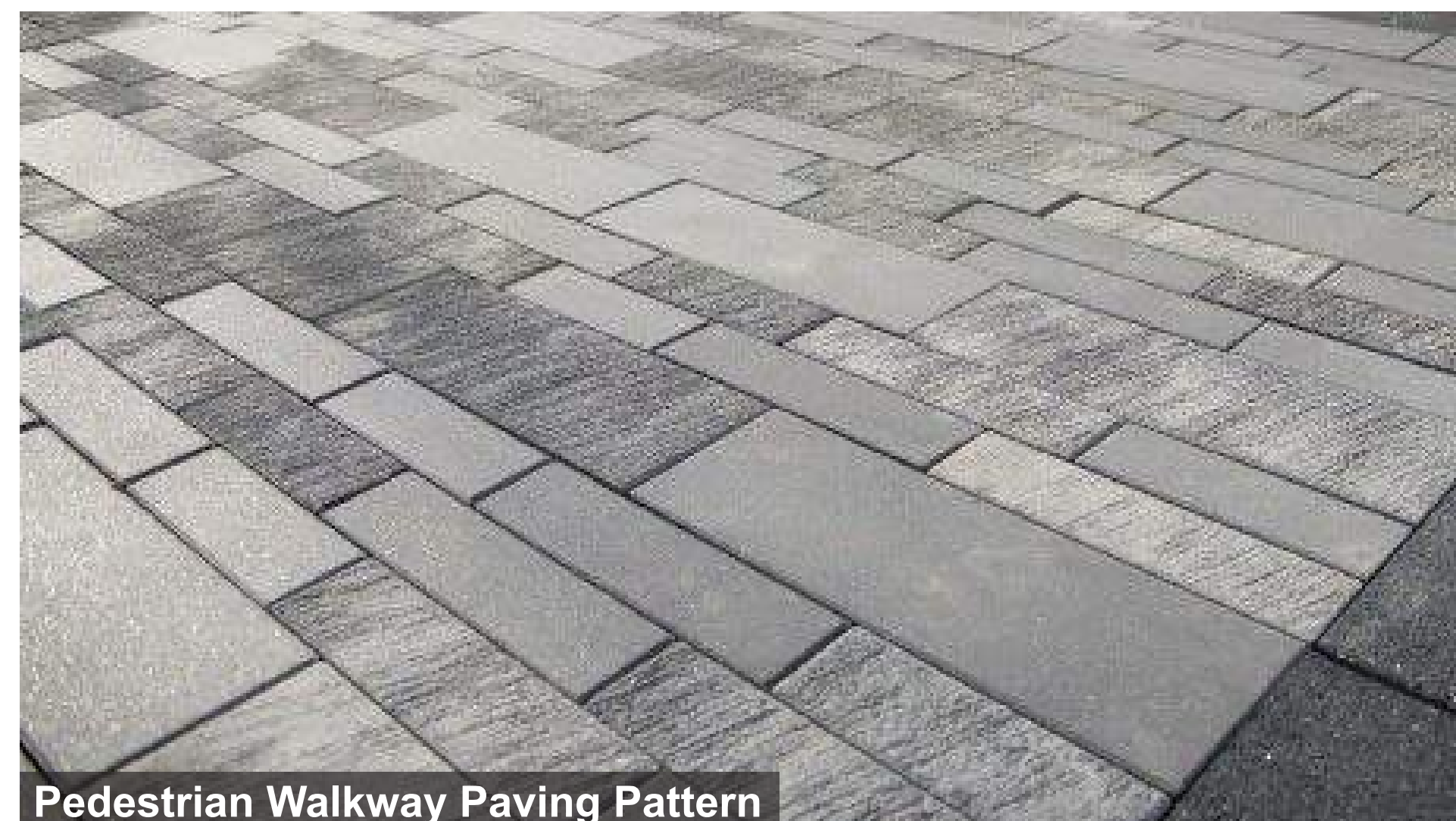
Pedestrian Walkway Paving Pattern
