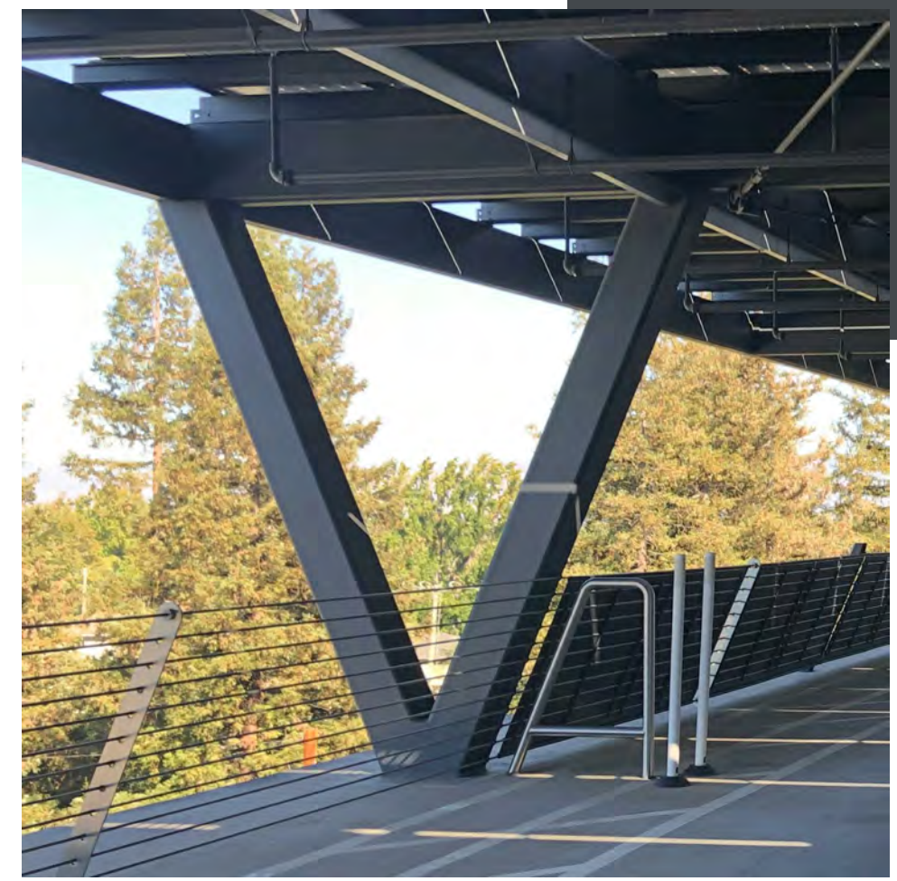
STEEL BRACE PARKING GARAGE STRUCTURE (MTL5) TYPE: METAL PRODUCT: STRUCTURAL BRACE COLOR: RAL 7024 GRAPHITE GREY PROTECTED FINISH: PAINTED
