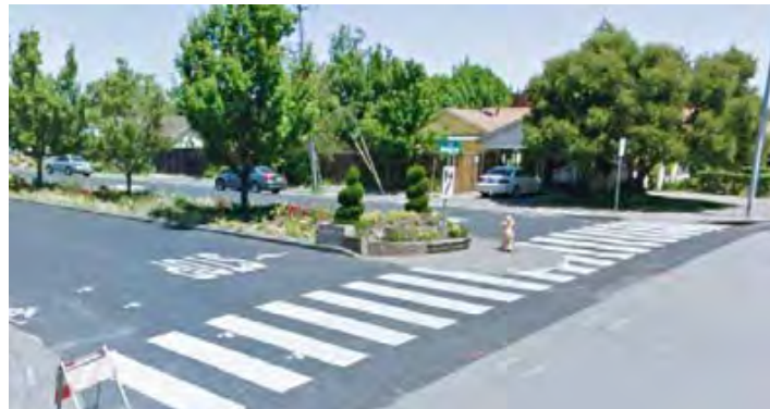
Install/upgrade pedestrian crossing (with enhanced safety features)
