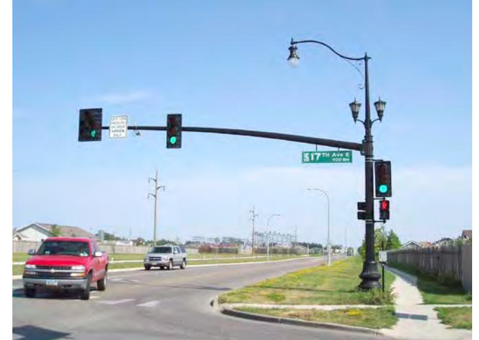
Convert signal to mast arm
