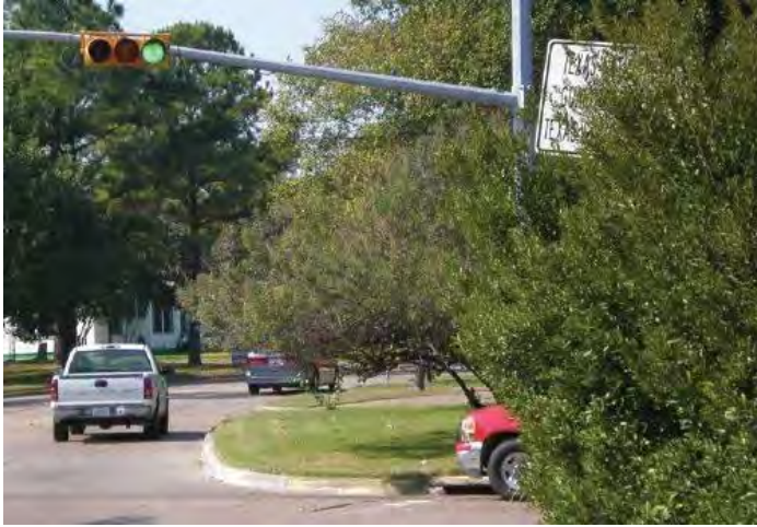
Improve sight distance
