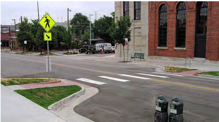
Install/upgrade pedestrian crossing (with enhanced safety features)
