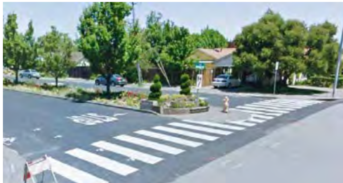
Install/upgrade pedestrian crossing (with enhanced safety features)
