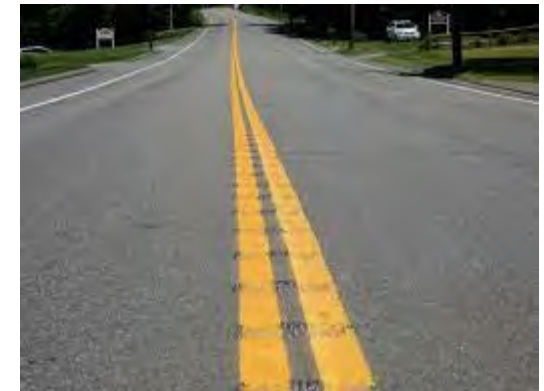
Install centerline rumble strips
