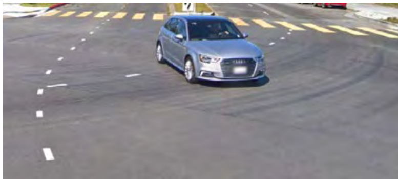
Install raised pavement markings
