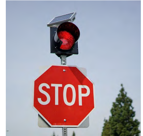
Install flashing beacons as advance warning
