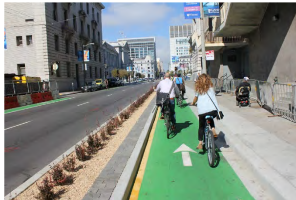
Install Separated Bike Lane
