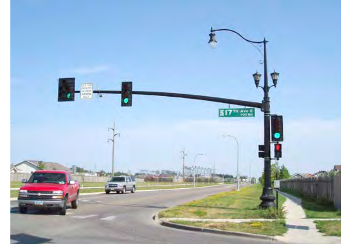
Convert signal to mast arm
