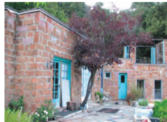
Woodhills Estate Cupertino/Saratoga Hills, End of Prospect Road – Mid-Peninsula Regional Open Space District, National Register of Historic Places
