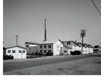
Woelffel Cannery 10120 Imperial Avenue Demolished
