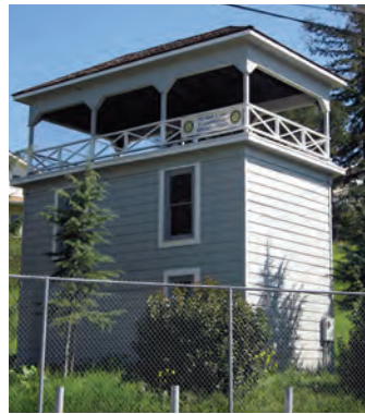
Nathan Hall Tank House 22100 Stevens Creek Blvd.
