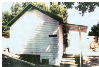
Montebello School 15101 Montebello Road
