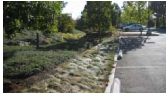
Parking lot runoff drains to a detention basin in Palo Alto.
