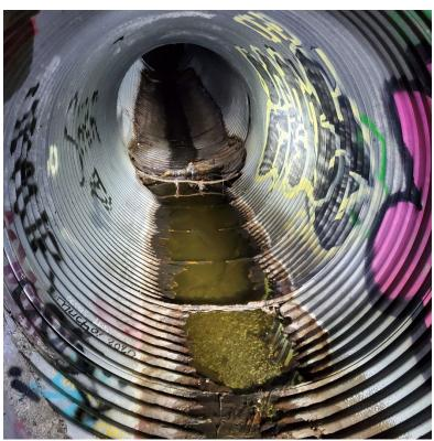
Photos of failed  $54^{\prime\prime}$  CMP storm drain main (September 2024):
