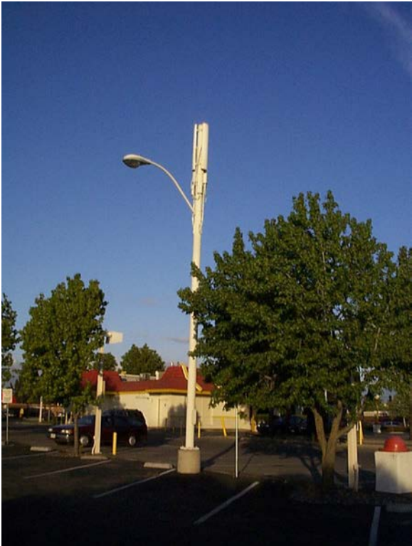
(Personal wireless service facility antenna/parking light standard pole in a shopping center off Highway 680, Pleasanton, CA.)
