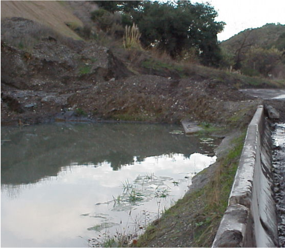
Pond 9 – from discharge looking East
