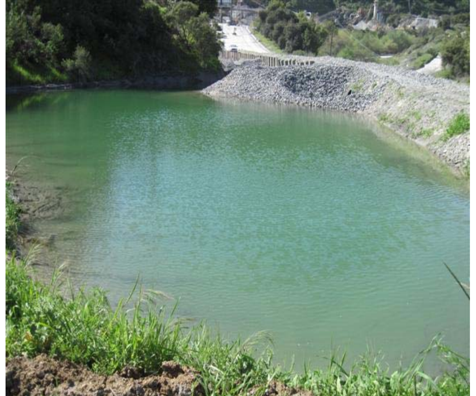
Pond 17 – looking last section before discharge
