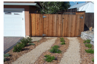
Wheel track driveway with gravel pavement
