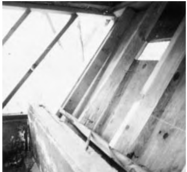
This photograph shows an interior detail of a home similar to the one at the left, showing substantial damage to a building with an unbraced tall wall.
