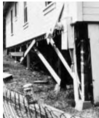
The pier-and-post foundation under this home shifted during a recent earthquake.
