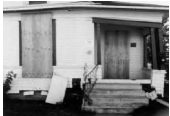
This home wasn't bolted and slid off its foundation.
