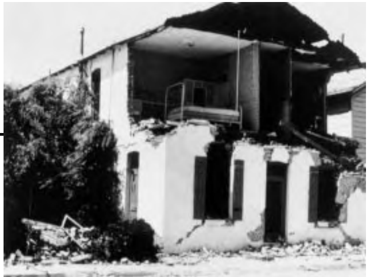
The plaster-covered brick walls of this building collapsed during a recent earthquake.
