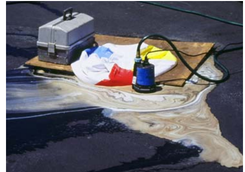
Storm drain inlet is blocked to prevent prohibited discharge. The water must be pumped and disposed of properly.
