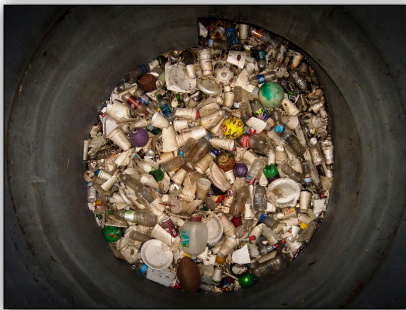
Photo 3: Lighter Materials in a Hydrodynamic Separator within the San José Storm Drainage System
