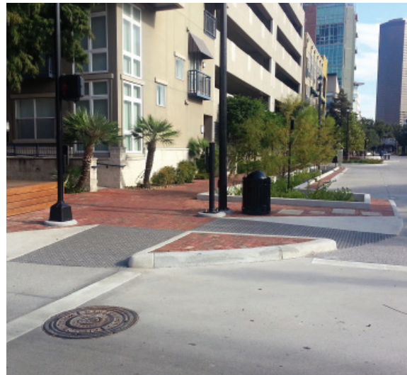
Bulbouts at street corners create shorter crossings for pedestrians and increase public space for landscaping, seating, and other amenities.
