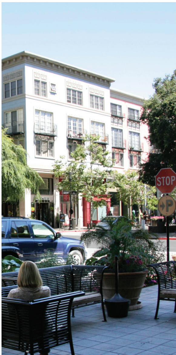
A redesigned shopping district will create a dynamic, pedestrian scale “downtown” in South Vallco
