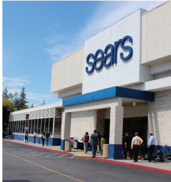
Many areas in South Vallco have limited sidewalks that were designed primarily to access stores
