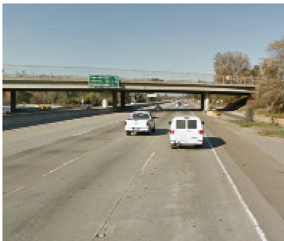
Interstate 280 provides great regional access to the South Vallco area
