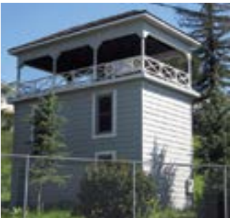
Nathan Hall Tank House 22100 Stevens Creek Blvd.
