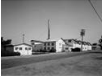
Woelffel Cannery 10120 Imperial Avenue – Demolished
