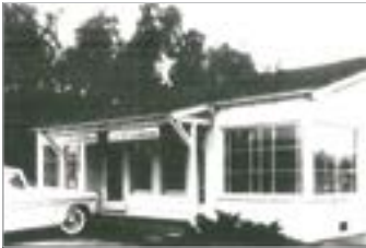
Interim City Hall 10321 South De Anza Boulevard
