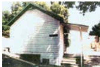
Montebello School 15101 Montebello Road
